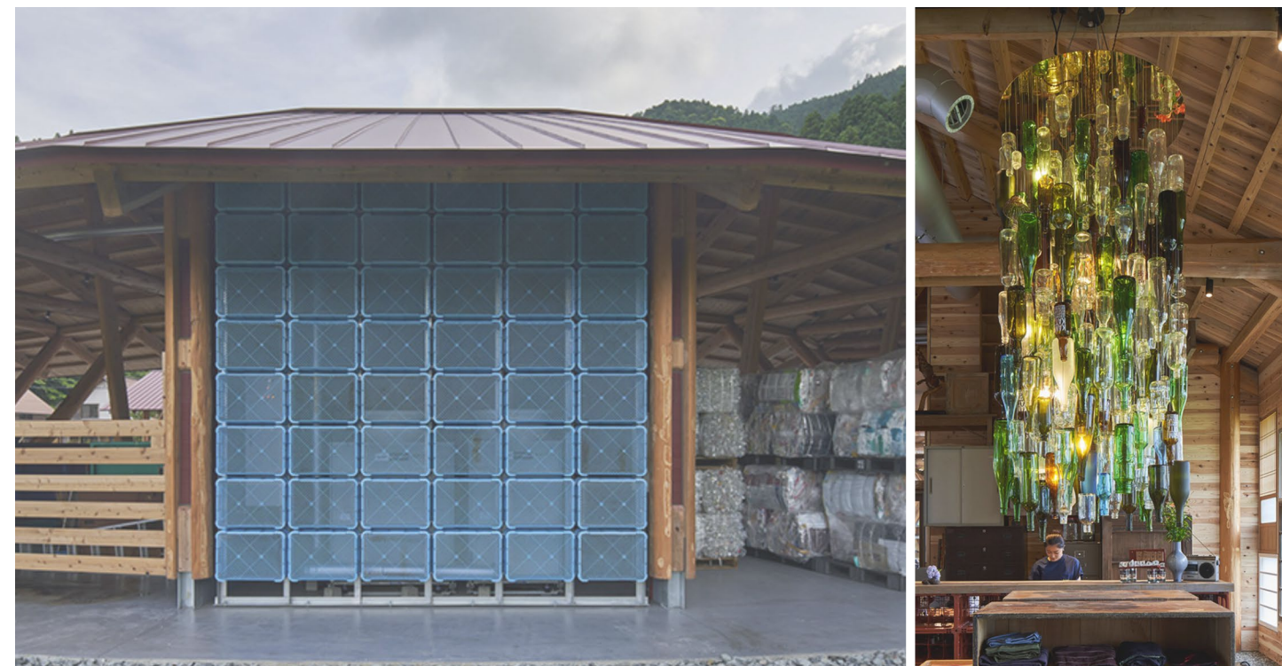
Figure 16. Plastic Tray Wall & Bottle Chandelier at Zero Waste Center. (photo by Koji Fujii / TOREAL)
