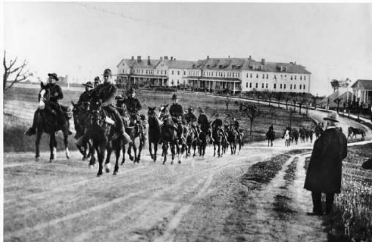
Figure 14. Oregon Avenue and the Parade Ground - with Gymnasium (right) and Double Barracks (demolished) (1914)
