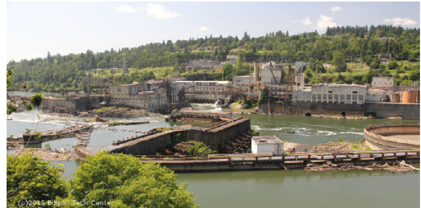
Figure 8.6: Willamette Falls hydroelectric dam, 2015. (Edison Tech Center)
