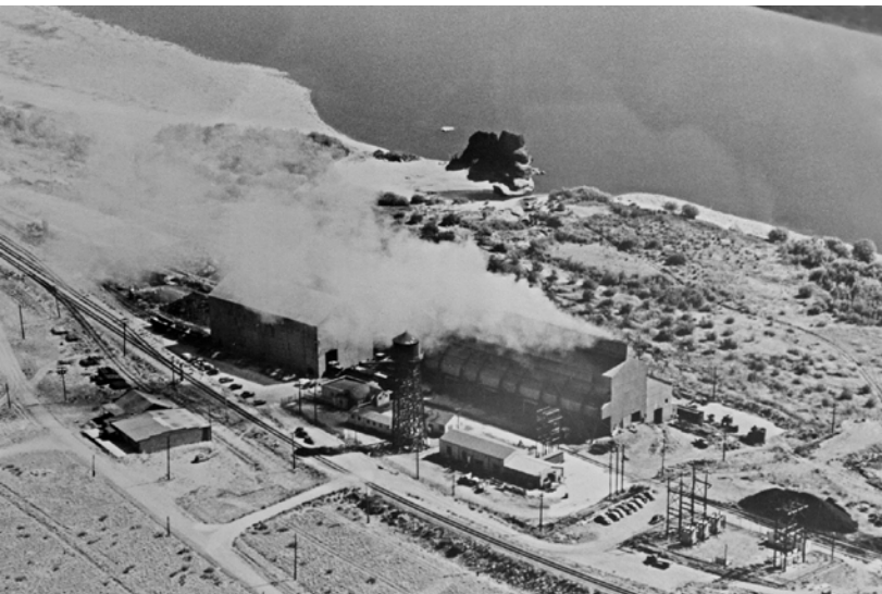
Figure 3.10: The smelter releasing silica fume into the air, 1955. The orchard and soft river bank can be clearly seen behind the buildings. (Big Bend Railroad History)
