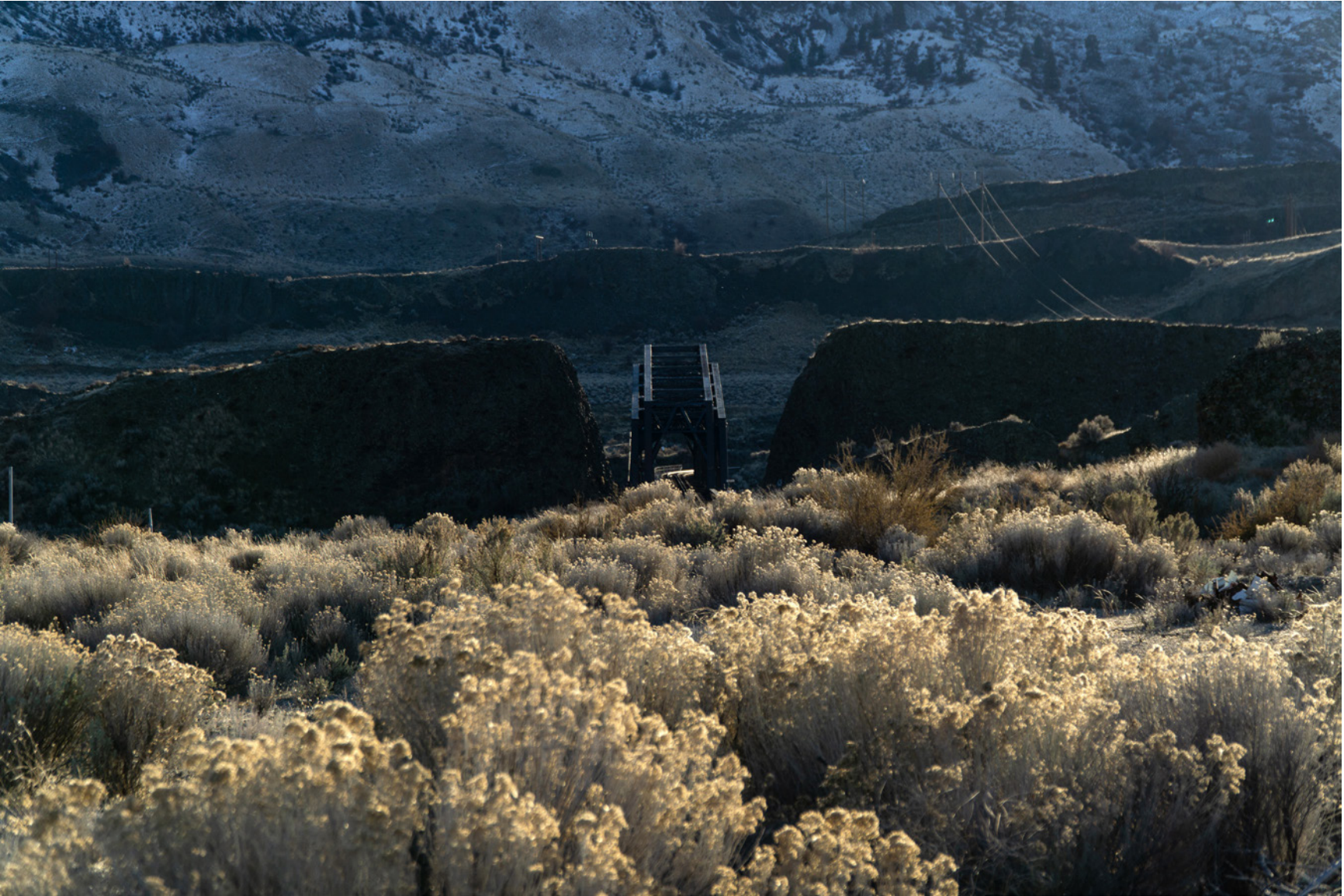
Figure 9.8: Looking south across the rabbitbrush covered slope toward the railroad bridge, from the Rail Overlook node.
