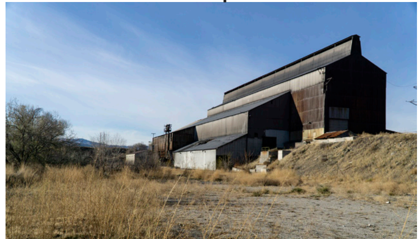
Smelter buildings, November 2018.
