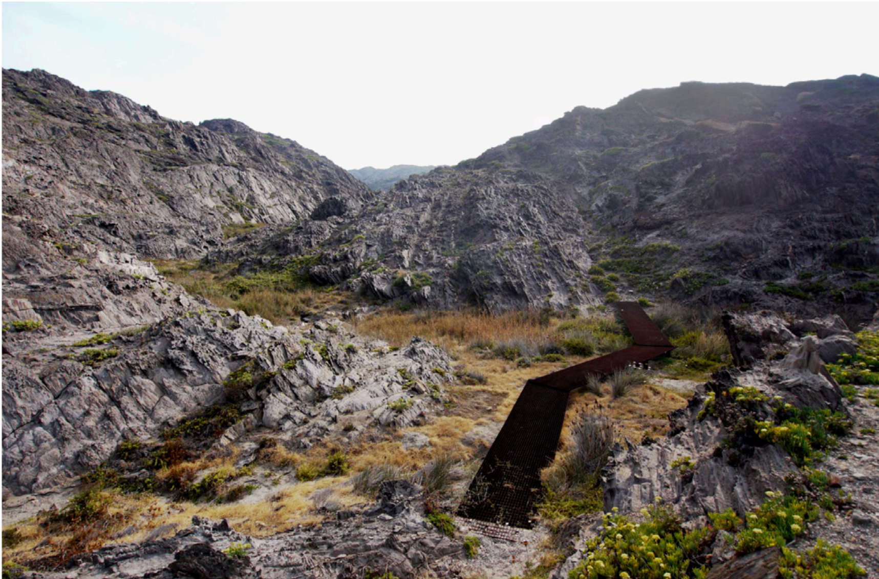
Figure 8.5: A steel grate elevated path. (EMF)
