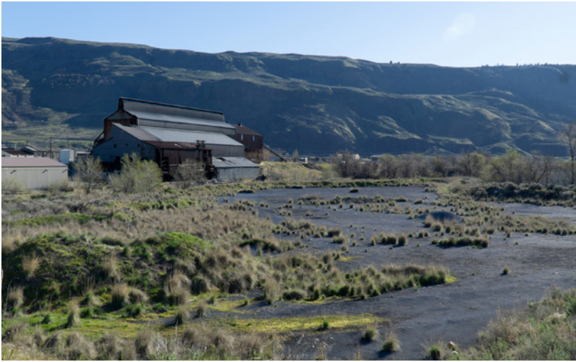
Figure 1.1: Silicon plant and silica fume waste ponds in April 2019.
