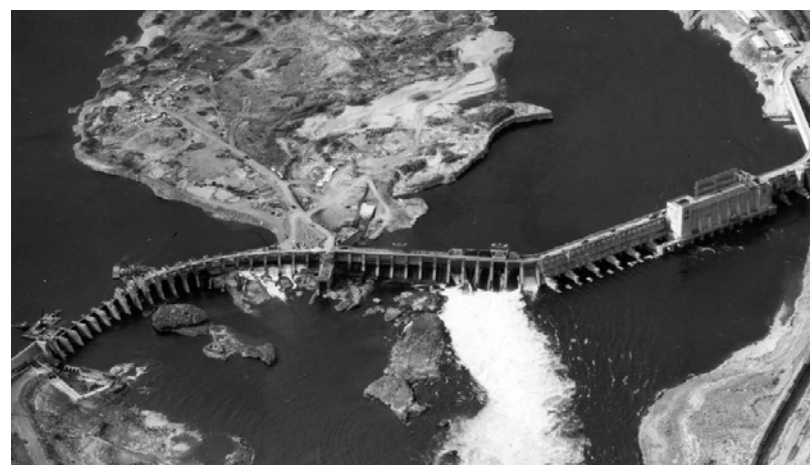
Figure 3.4: Rock Island Dam c.1950. (Chelan County PUD)
