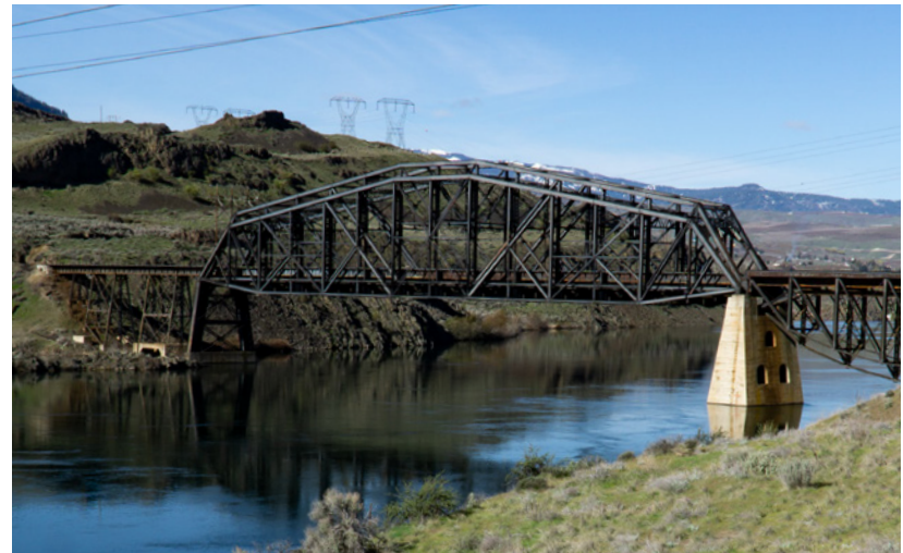
Figure 3.6: Rock Island railroad bridge. April 2019.
