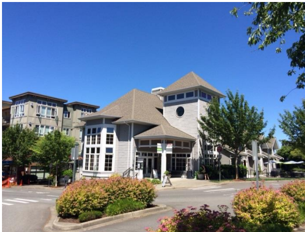
Figure 13 Blakely Hall Community Center
