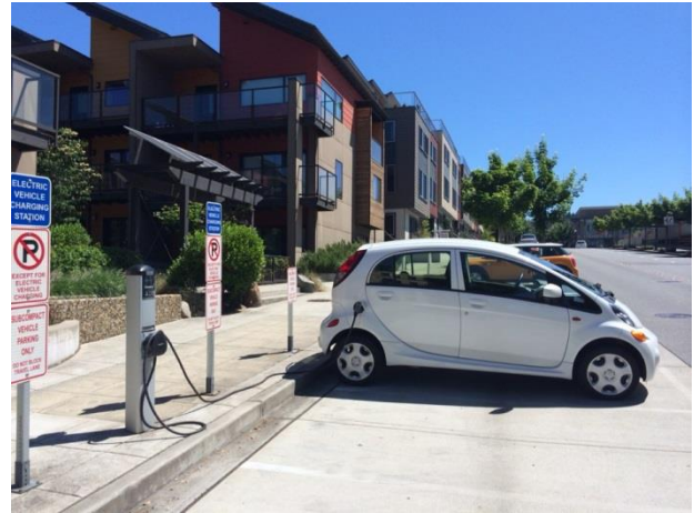
Figure 16 Electric Charging Station at zHome
