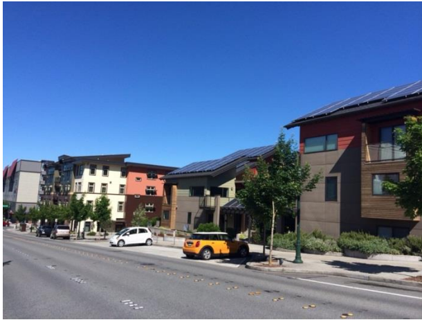
Figure 15 Solar Energy System at zHome
