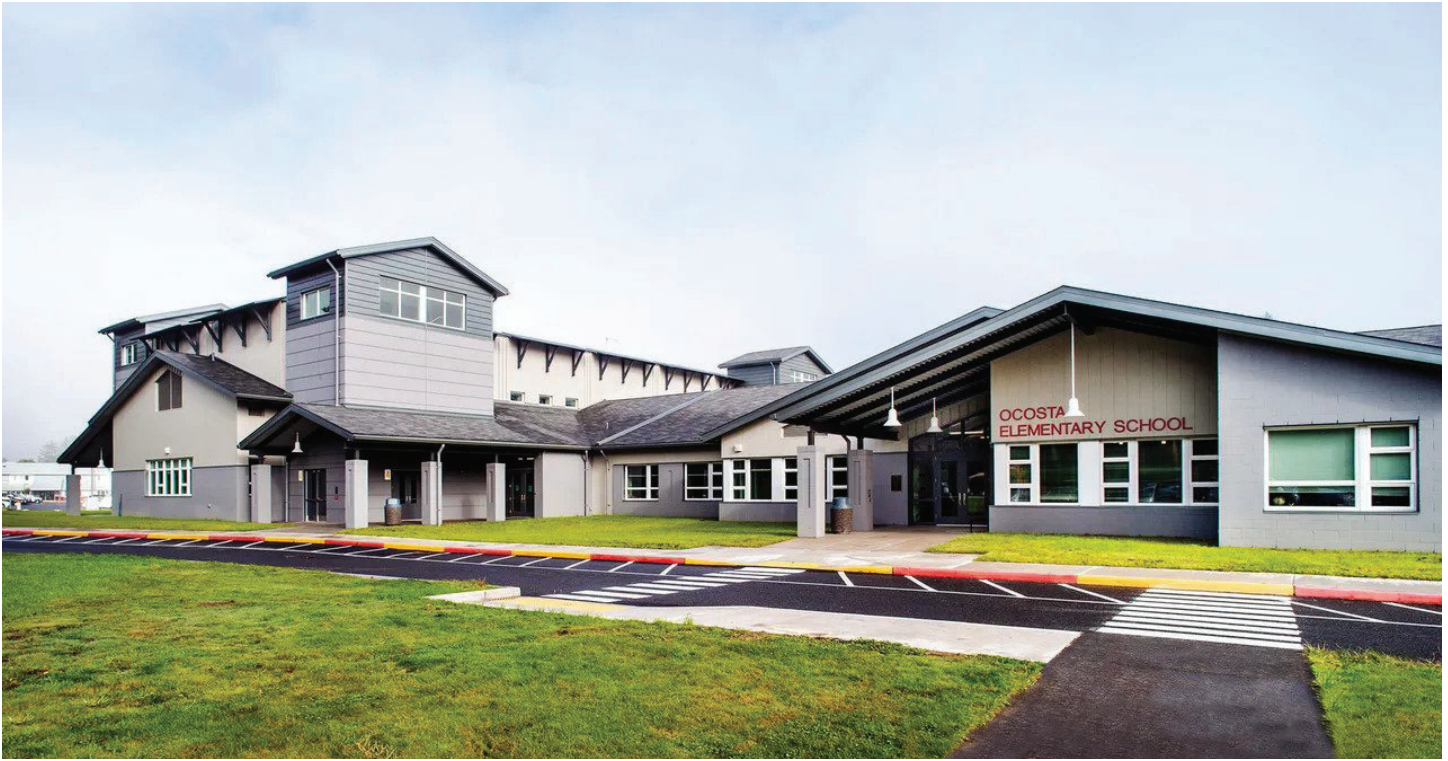
Figure 4.16: Ocosta Elementary School Source: Wired Magazine
