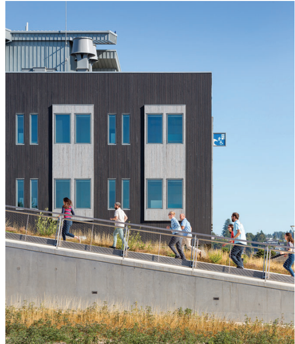
Figures 3.10: Users climbing the ramp to the rooftop VES. Source: Josh Partee
