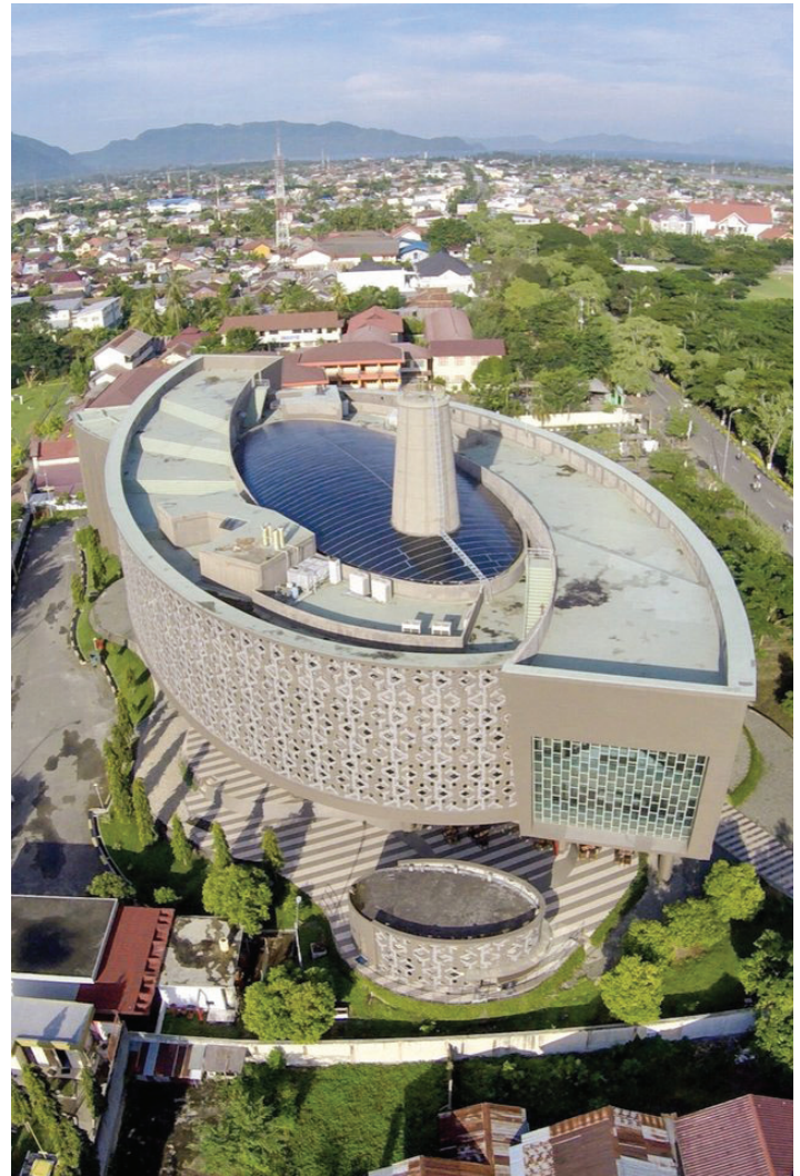
Figures 3.8: The rooftop VES in Banda Aceh. Source: Abdul Hadi
