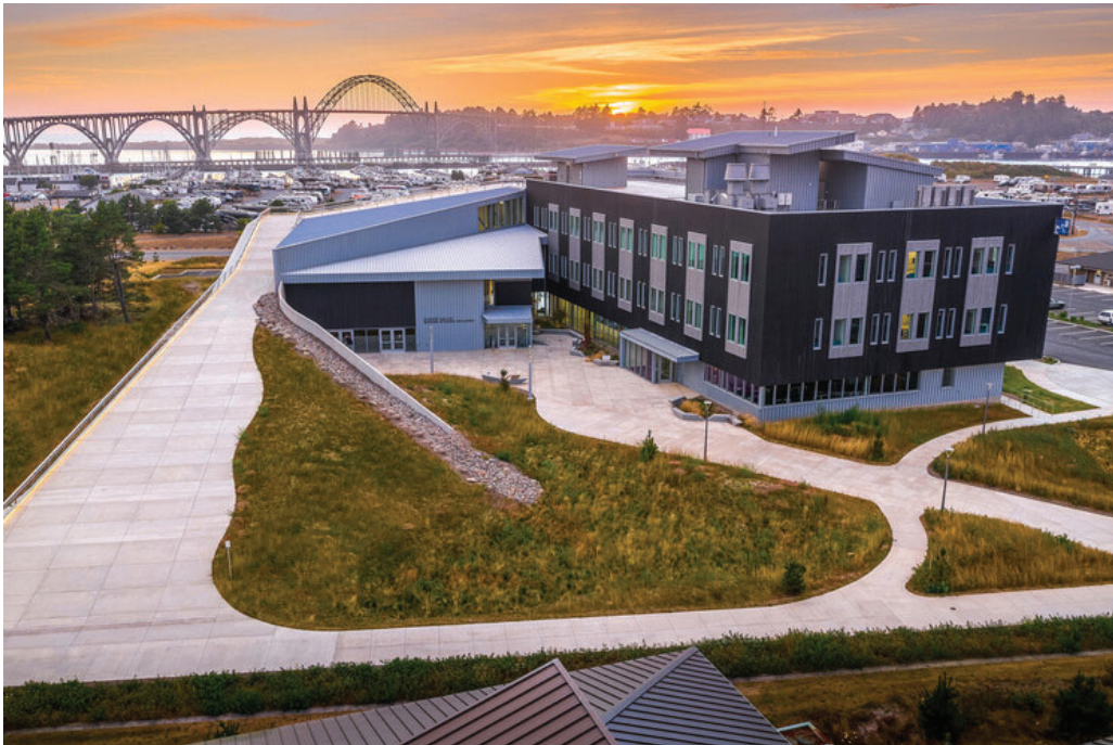
Figures 3.9: The ramp leading to the VES on the roof. Source: Josh Partee
