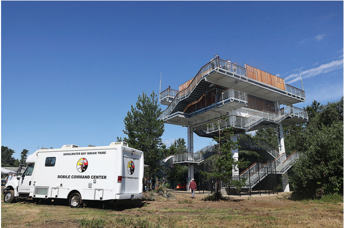
Figures 3.6: The new VES on the Shoalwater Bay Tribe land. Source: Washington Military Department
