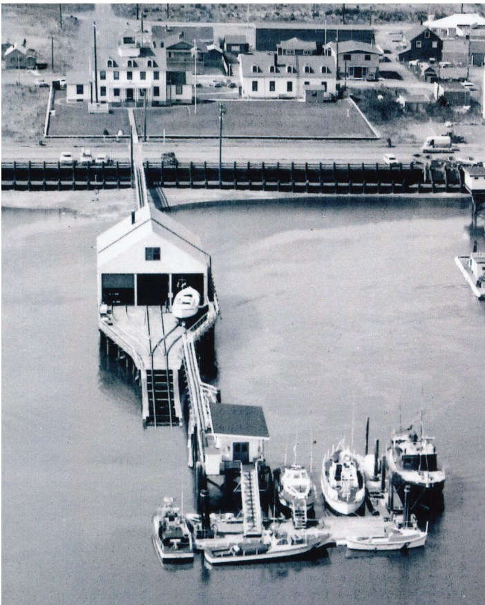
Figure 4.13: The historic boathouse to be replicated on site. Source: Westport Maritime Museum
