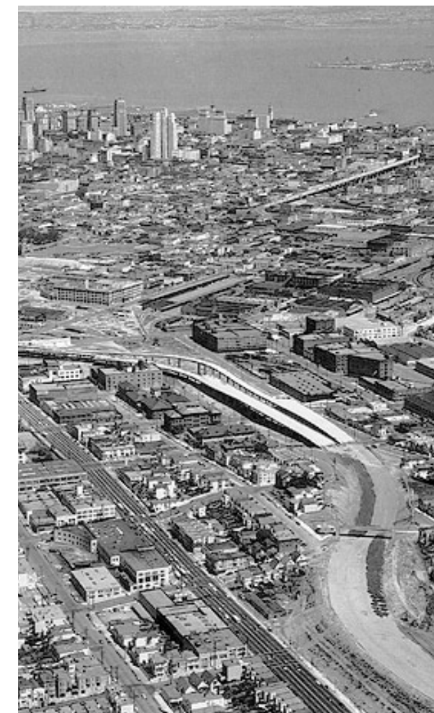
Image_ James Lick Freeway under construction. Found SF : Ed Brady (1953).
