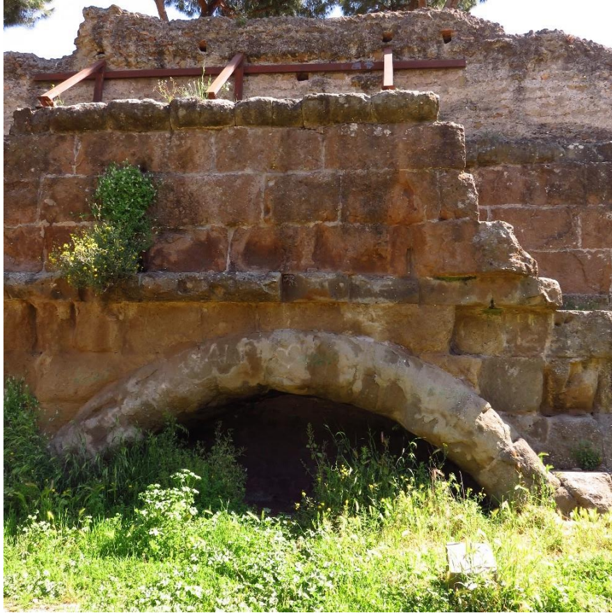
Figure 1.1. Arcade of the Aqua Marcia in the Parco degli Acquedotti, Rome. Spandrels of light, soft tufa; rings of arches and projecting slabs of grey peperino; channel walls of reddish-brown tufa.
