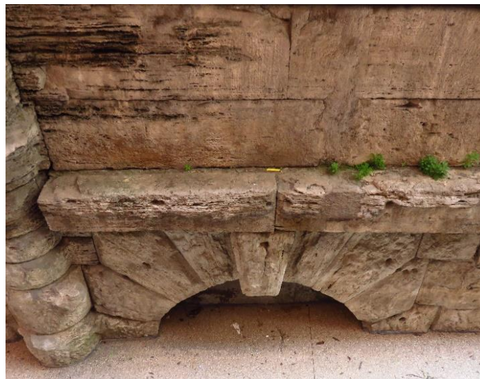
Figure 1.9. Preserved upper portion of the arcade of the Aqua Virgo which led to the aqueduct's terminus near the Pantheon (cf. Figure 1.6 f). Maximum height of the arcade c.10m. Peperino and travertine. Near intersection of Via Nazzareno and Via del Tritone, Rome.
