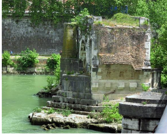
Figure 1.20. The Pons Aemilius (“Ponte Rotto”).
