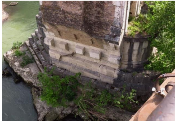
Figure 1.21. Detail of (Augustan?) flood protection on the Pons Aemilius.
