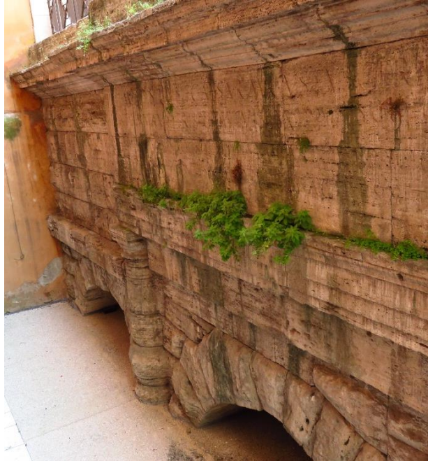
Figure 1.8. Preserved upper portion of the arcade of the Aqua Virgo which led to the aqueduct's terminus near the Pantheon (cf. Figure 1.6 f). Maximum height of the arcade c.10m. Peperino and travertine. This arcade dates to a Claudian rebuild of 46 CE, recorded in the inscription over the arch (foreground) which spanned a roadway ( ILS 205 = CIL 1252). Near intersection of Via Nazzareno and Via del Tritone, Rome.
