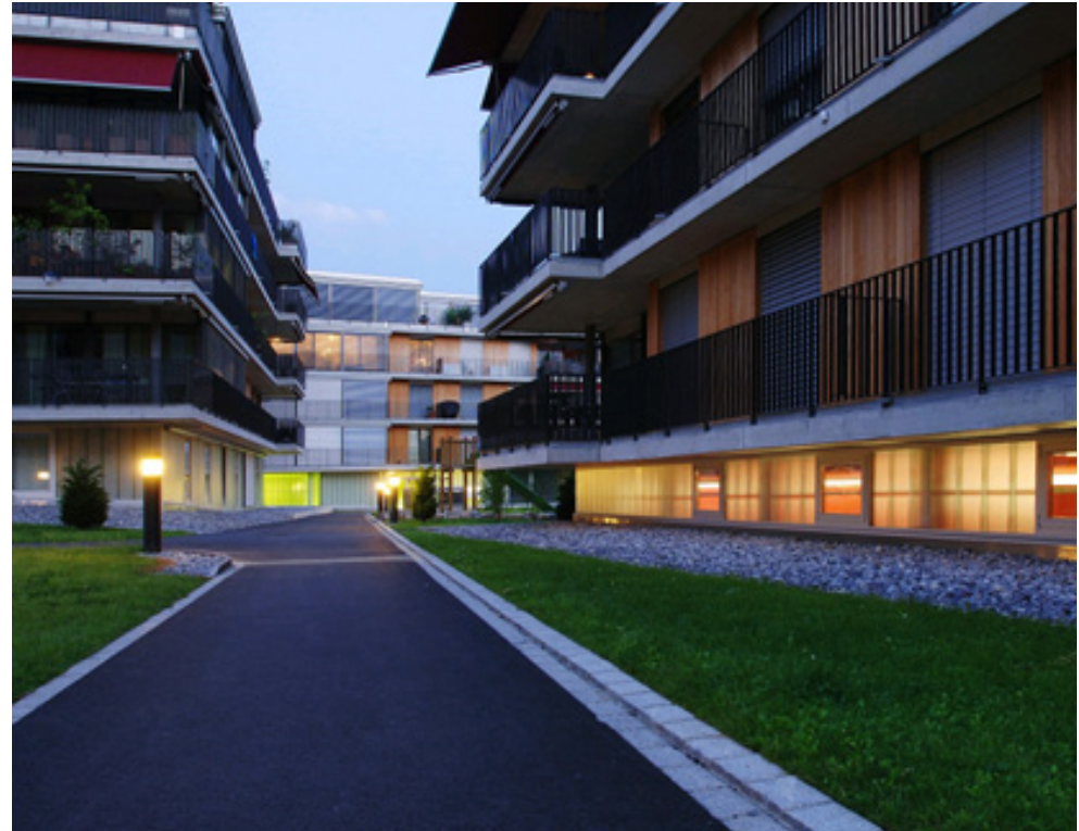
Figure 26: Intergenerational Housing in Europe Image: http://blog.buildllc.com/wp-content/uploads/2010/03/Wohnu-berbauung-Steinacker-01.jpg (Accessed Sept 11, 2015)
