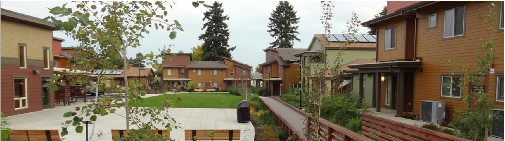
Figure 27: View of Courtyard Image: Bridge Meadows (Home), http://www.bridgemeadows.org (Accessed Sept 11, 2015)
