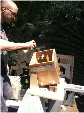
6. applying release agent : PAM
