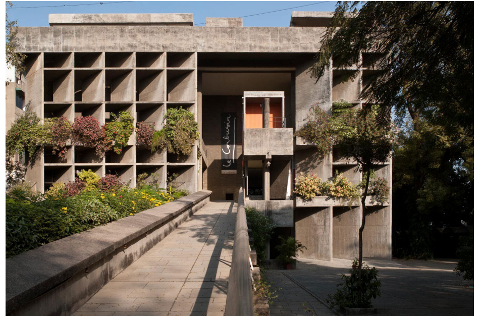
[fig. 30c] Ahmedabad Textile Mill Owners' Association House (ATMA House), Ahmedabad, India
