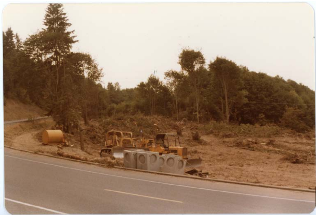
[Image 13] Making a ‘big hole,’ Johnson Pit #30 construction, 1979 (King County Archives).
