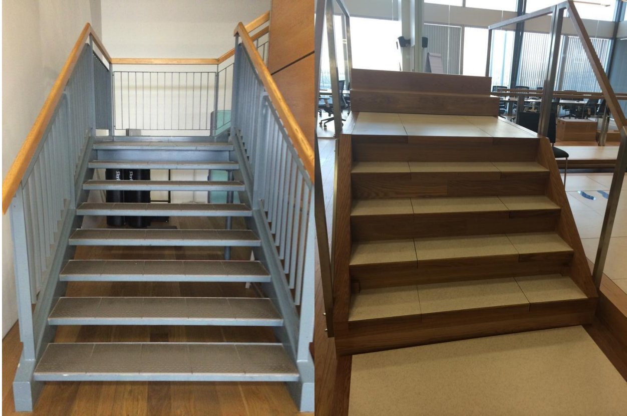
Figure 2.7: Staircase 1 on the left and staircase 2 on the right
