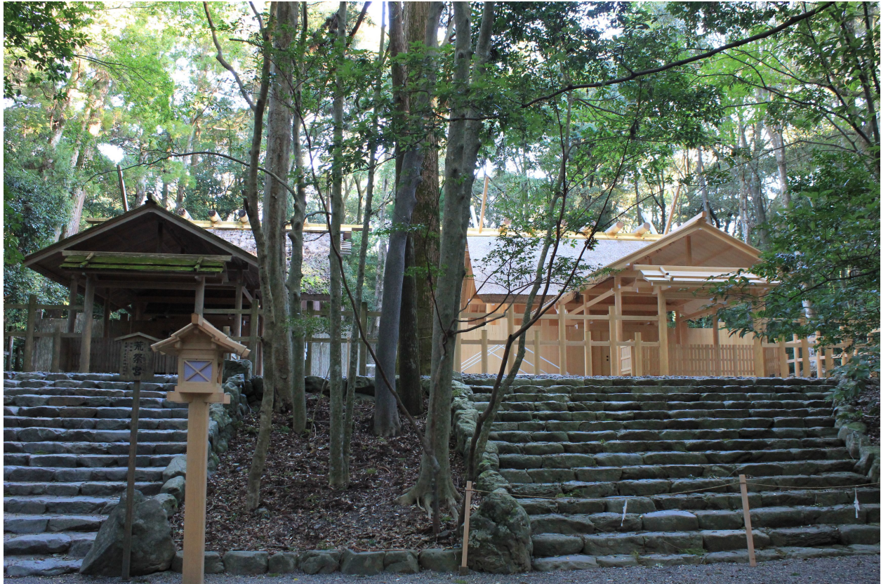
Figure 3: Newly built Aratsumirinomiya, one of the main auxiliary shrines of Kōtaijingū, at right and the old one at left. Soon after the enshrined deity had been transferred from the old one to the new one, the old shrine building was disassembled. (September 17, 2013)
