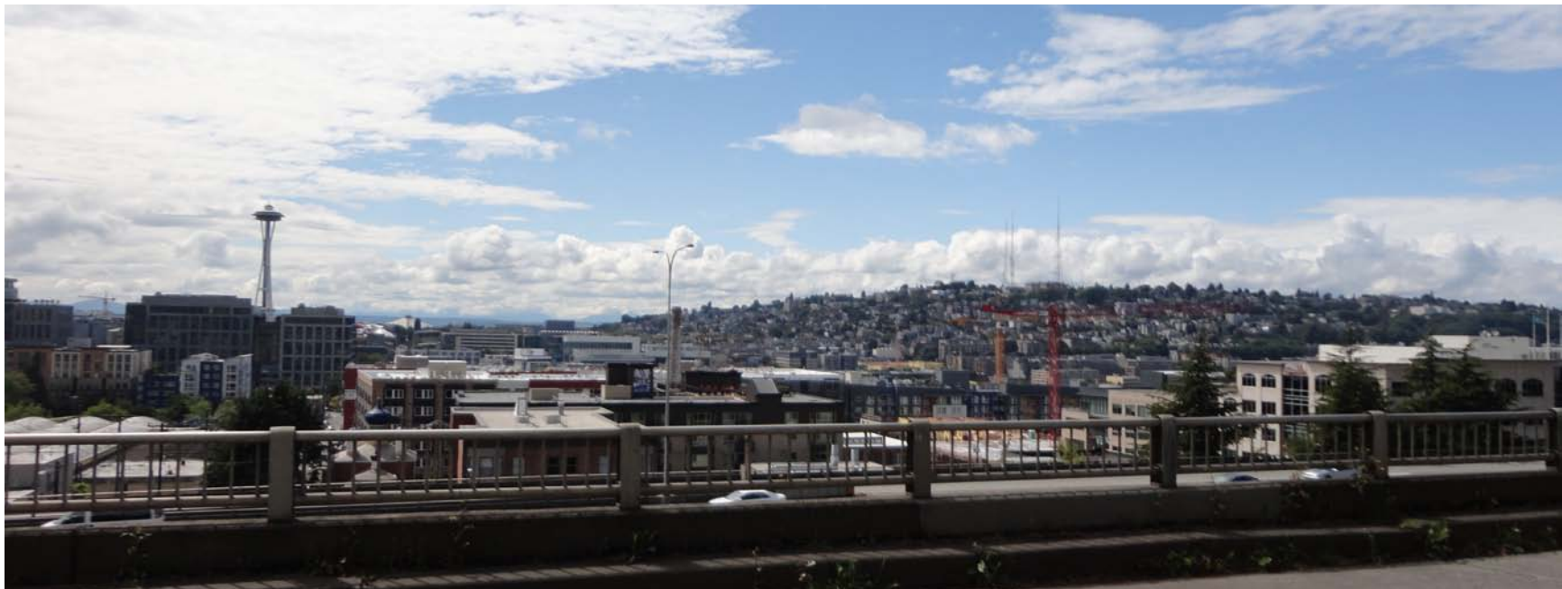
figure 21: View from the bottom of the Harrison pedestrian stair on the Melrose trail. The space made by the freeway allows for light and view that doesn't reach the denser areas of the city.
