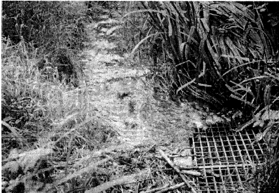
Figure 11. Ravenna Creek draining into the North Trunk Sewer.
