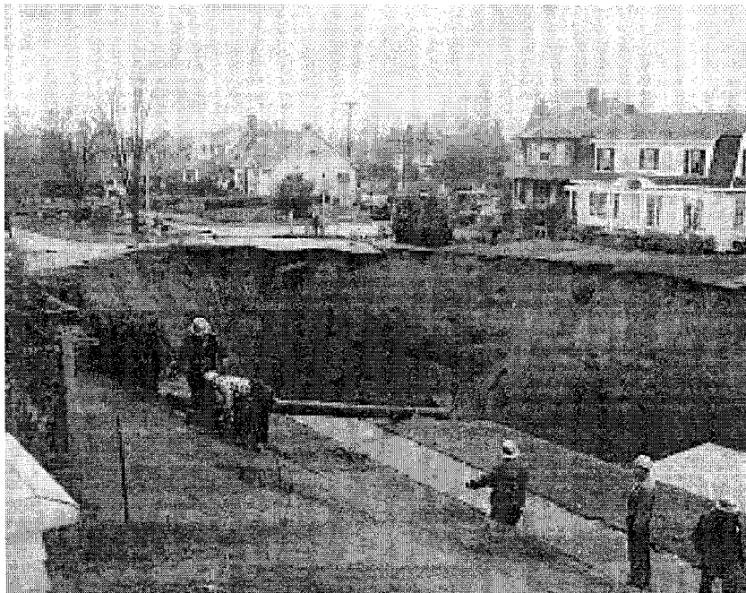
Figure 12. Sink hole caused by North Trunk sewer line break, Seattle, ca 1957. Museum of History & Industry Photograph Collection, PI24322
