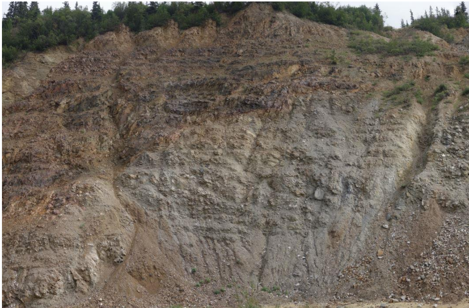
Figure 2.5 Slope at parks highway showing the darker volcanic rock, on top of the lighter Healy schist.
