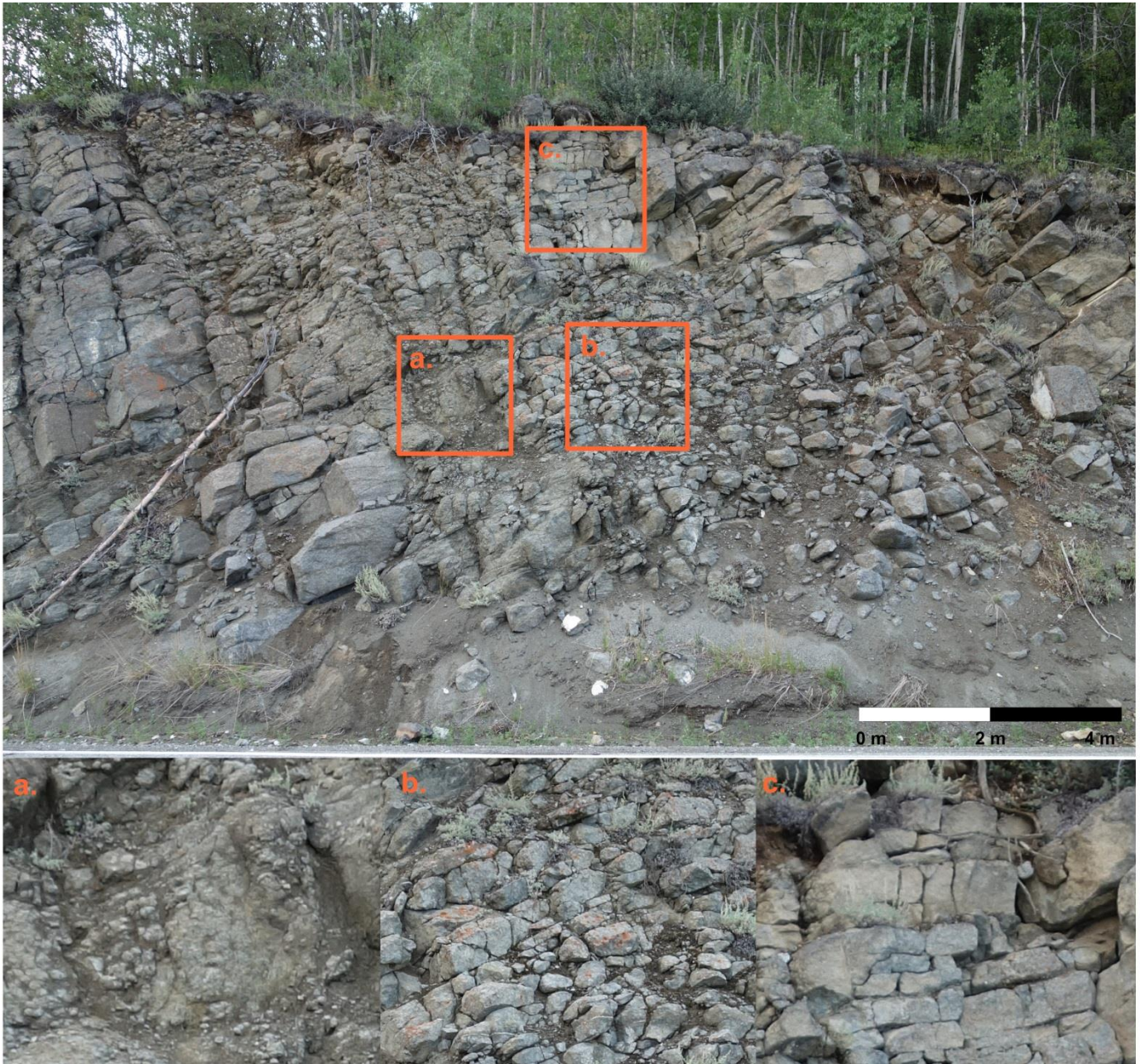
Figure 6.3: Examples of 10 cm, 20 cm and 30 cm active classifications for the RAI at milepost 85
