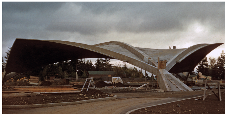
Figure B.2: Construction photo of auditorium showing primary reinforced concrete structure
