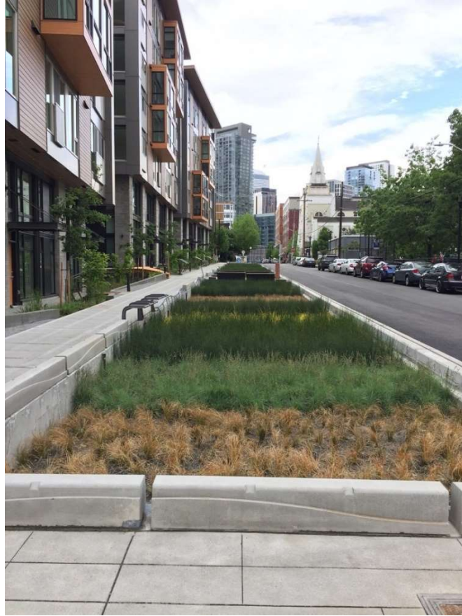
Figure 10: Swale on Yale along Pontius Avenue. Innovation in sustainable urbanism. Picture taken 5/17/2019.
