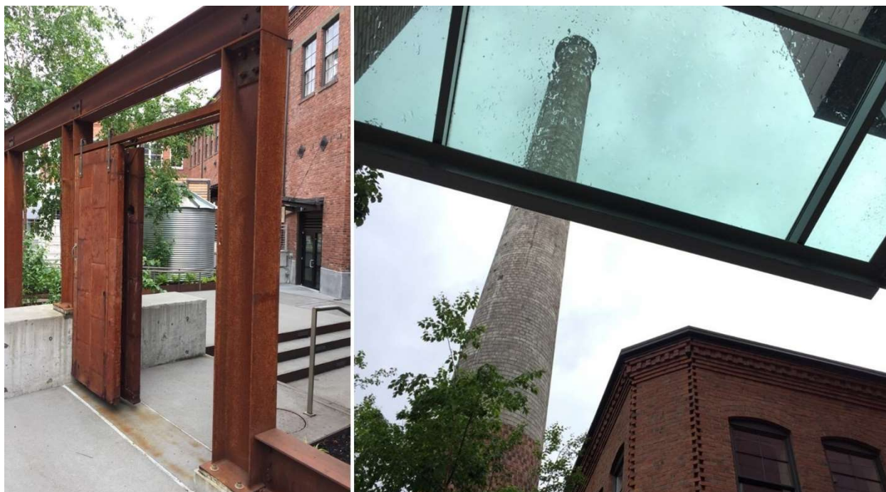
Figure 14: The 2014 Stack House apartment complex on Harrison Street includes office and restaurant space in the 1904 Supply Laundry building (registered in the National Register of Historic Places 38 ), of which the brick facades, timber beams and wooden windows have been preserved. The laundry’s masonry smokestack is the centerpiece of the complex’s courtyard and advertised as “a touchstone of a bygone era” 39 . Pictures taken 6/3/2019.
