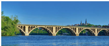
FRANCIS SCOTT KEY BRIDGE
