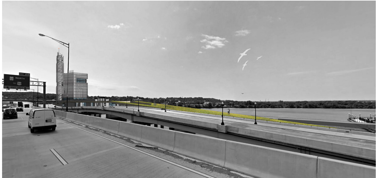
Fig. 72: The project as seen from I-695 bridge
