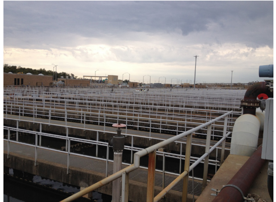
Fig. 33: Blue Plains Wastewater Treatment Plant
