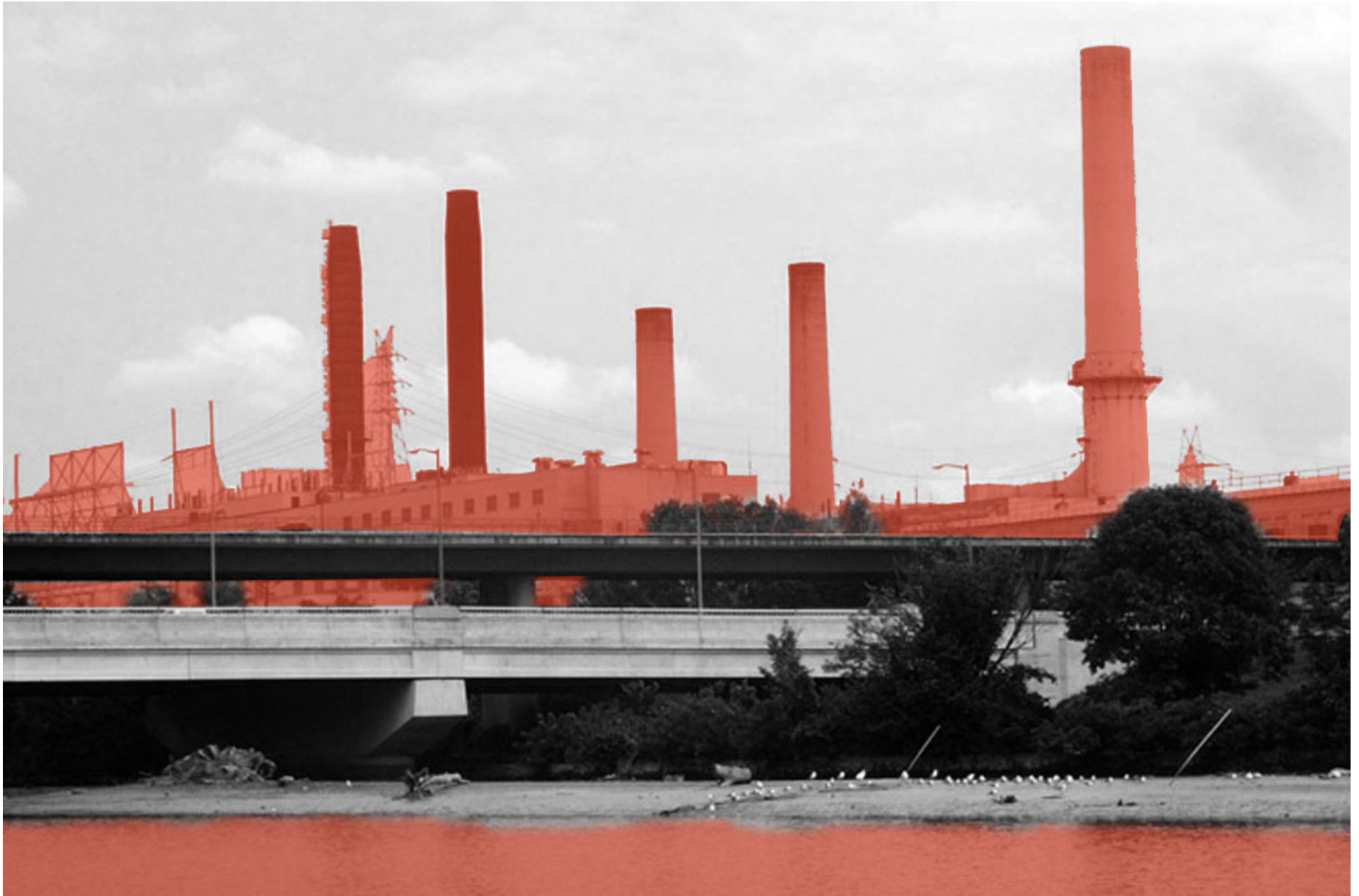
Fig. 20: Benning Road Power Plant with Anacostia River in foreground
