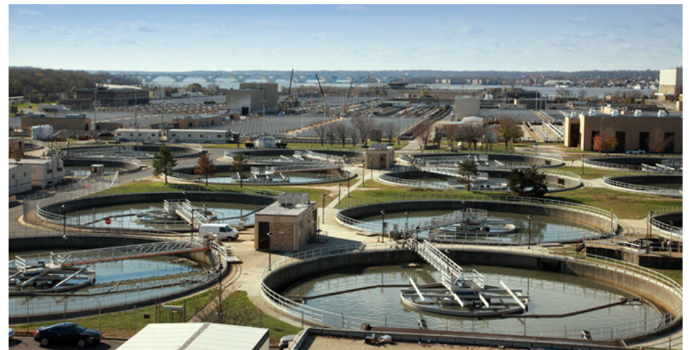
Fig. 34: Blue Plains Wastewater Treatment Plant, Source: aecom.com
