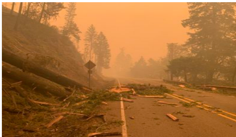
Figure 4.2: Photos of damage in the Susan Creek area by ODOT [40]
