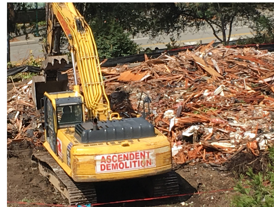
Fig. 49 - Demolition 1 Fig. 50 - Demolition 2
