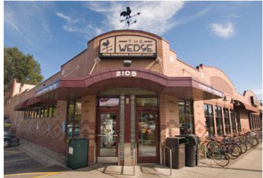
Image 9 : Exterior View of The Wedge
