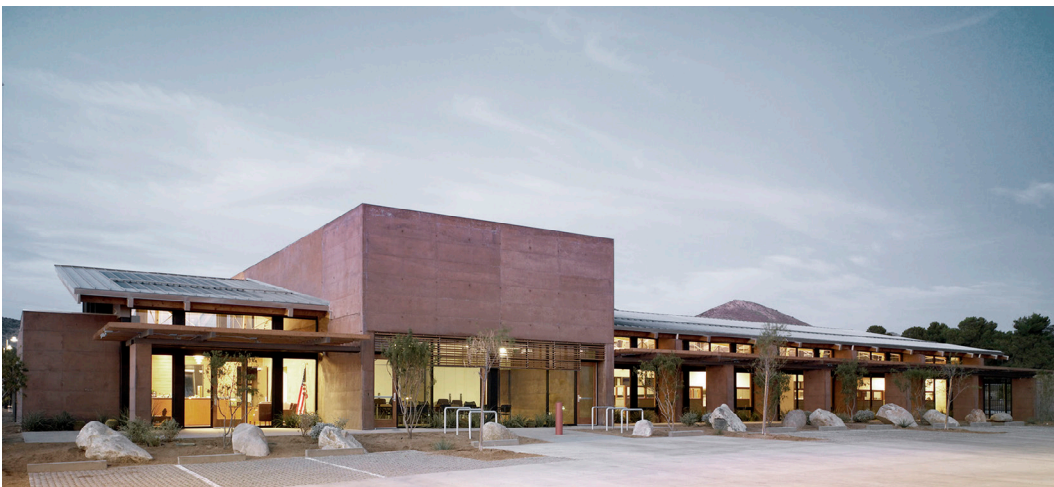
fig. 73 - The tinted concrete wall reflect the surrounding tone of the Sonoran Desert. fig. 74 - A trellis and sunshade block summer heat gain and create semi-sheltered outdoor space. fig. 75 - The massing divides the ranger station into three areas based on interior program.
