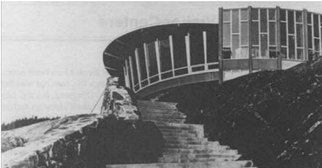
fig. 34 - CCC built Chelan Ranger Station on the Wenatchee National Forest fig. 35 - CCC built fire lookout on the San Juan National Forest - 1939 fig. 36 - Picnic shelter built by the CCC shows off rustic log construction fig. 37 - CCC built ranger station on the Bighorn National Forest - 1938 fig. 38 - Mendenhall Glacier Visitor Center on the Tongass National Forest - 1961
