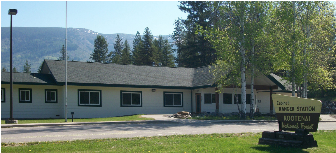
fig. 39 - Region 6 Forest Science Lab in Olympia, Washington - 1967. fig. 40 - Colville National Forest Headquarters in northeastern Washington. fig. 41 - Prefabricated concrete pit toilet bathroom, one of many across National Forests in the northwest. fig. 42 - Cabinet Ranger District on the Kootenai National Forest in western Montana.
