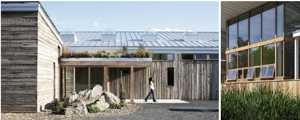
fig. 69 - Functional and amenity spaces are architecturally defined but still interact with each other. fig. 70 - The pitched roof directs water to the constructed wetland. Primary interior spaces view out to the wetland. fig. 71 - The building has a campus wide function but the front entrance is human scaled and features reclaimed wood. fig. 72 - Operable glazing increases occupant comfort.
