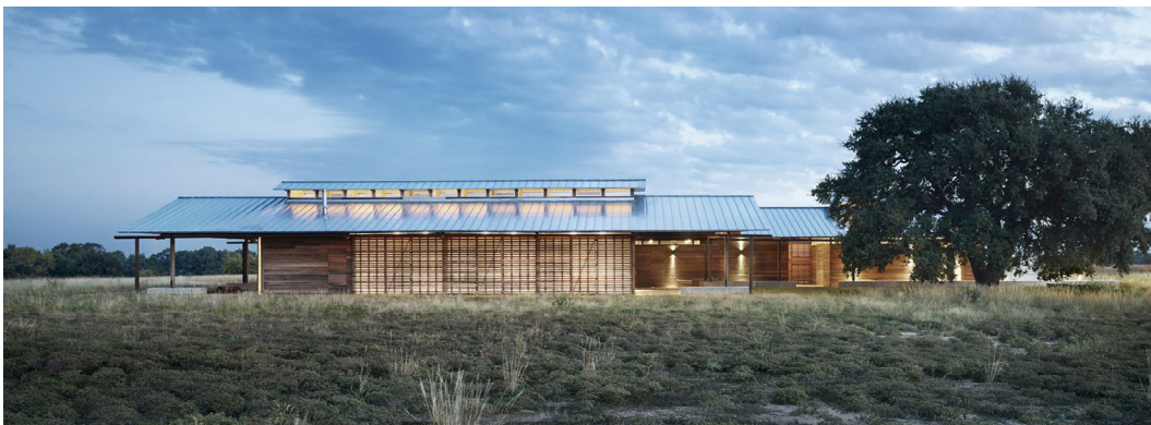
fig. 62 - Tillamook Forest Interpretive Center fig. 63 - Omega Center for Sustainable Living fig. 64 - Mojave Rivers Ranger Station fig. 65 - Dixon Water Foundation – Josey Pavilion
