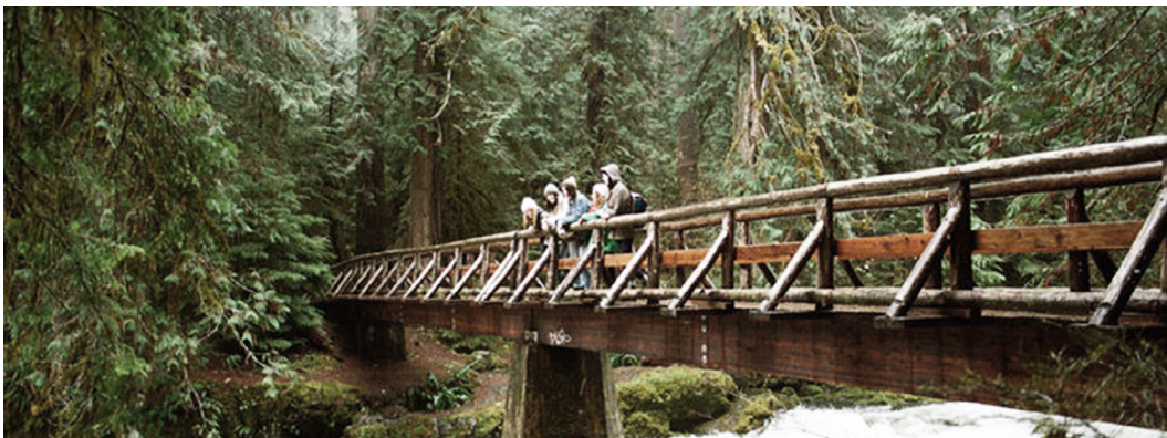
fig. 59 - Lakeside campsite with a view of the Sawtooth Mountains fig. 60 - Forest Service trail crew clear downed logs blocking a hiking trail fig. 61 - On a popular hiking trail, a bridge spans the river and eases travel
