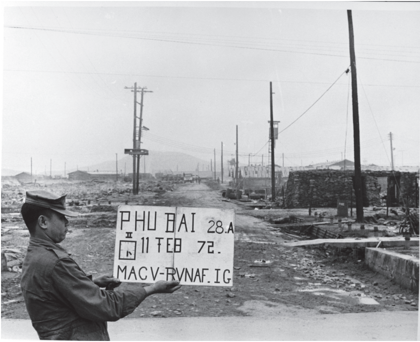
FIGURE I.1. Demolished troop billets at Phú Bài Combat Base, February 11, 1972. Source: Box 3, RVNAF Base Turnover Inspections, MACV Inspector General Records, Record Group 472, US National Archives and Records Administration, College Park.
