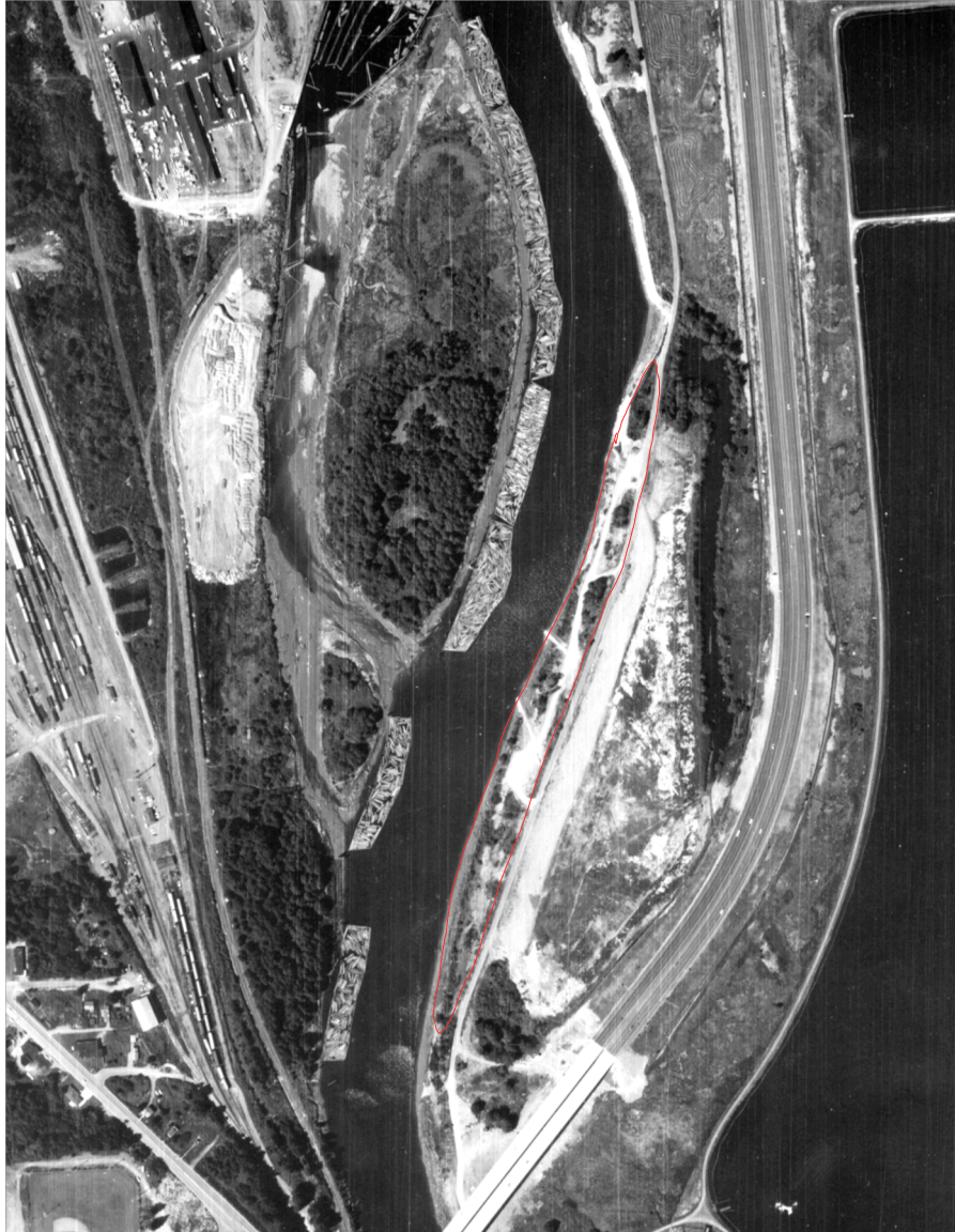
Figure 8: Aerial photograph of the park location taken in 1970.
