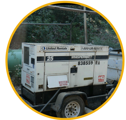
E. Barn Energy Hub
