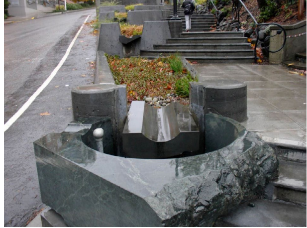
Figure 4.8: Runnel and rain gardens fed by roof runoff. (Credit: photo by Buster Simpson).
