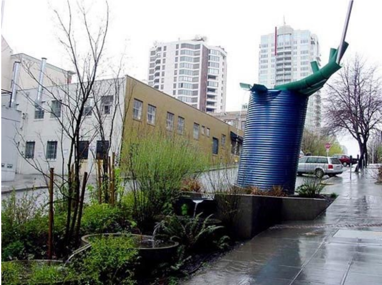
Photo 4.6: The Beckoning Cistern on Vine Street is fed by roof runoff from an adjacent building and is the beginning of a series of rain gardens along Vine Street which help to clean and irrigate streetscape plantings. A portion of the water collected also feeds a cistern for use in gardening. (Credit: photo by Buster Simpson).
