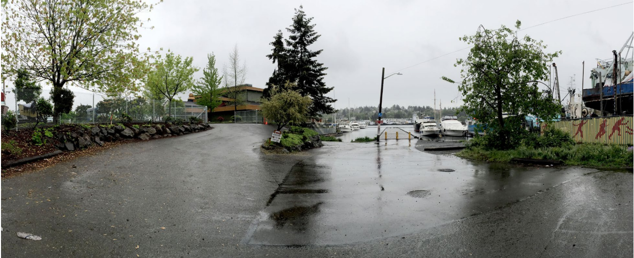
Photo 5.11: Panorama at 24th Ave NW street end, April 24, 2016. The defunct Yankee Bar & Grill building is visible on the left. Chain-link fencing around the existing parking lot is in place for the future construction staging for the Ship Canal Water Quality Tunnel Project. (Credit: Rhys van Bommel).
