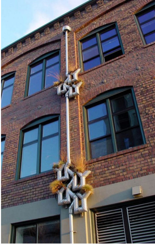
Photo 4.7: Sculptural planters incorporated into downspouts on a building on Vine Street. (Credit: photo by Buster Simpson).
