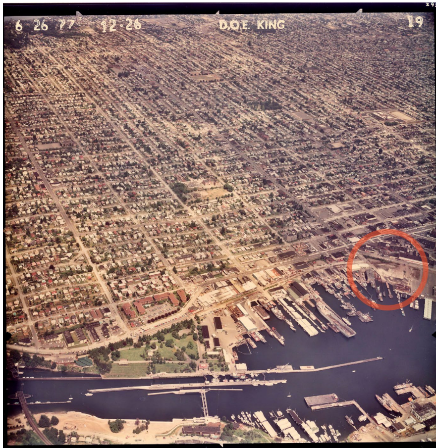
Photo 1.1: 1977 aerial of Hiram M. Chittenden Locks & Salmon Bay looking northeast. 24th Ave NW street and The Yankee Bar & Grill visible under construction in center right (circled). (Credit: King County Department of Engineering).
