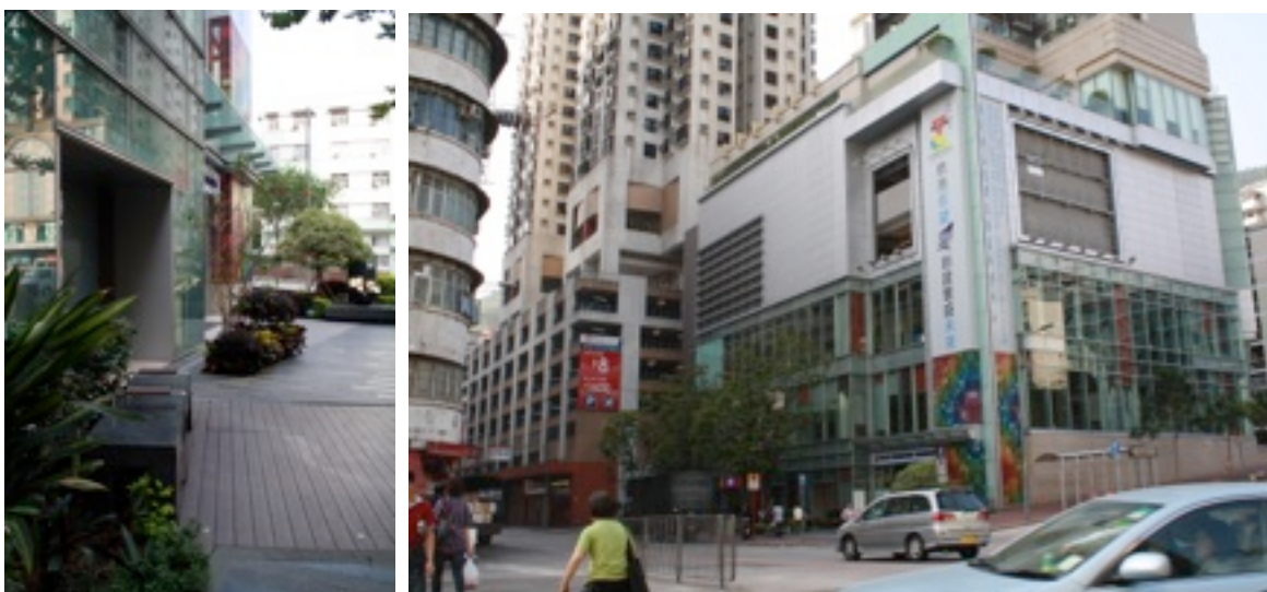
Fig 7.4 Beacon Lodge URA’s project in Sham Shui Po. The podium part is now owned and operated by YMCA as a private Lifelong-Learning center .
