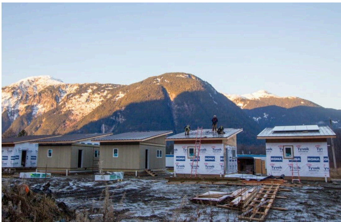
Figure 13. Nuxalk Tiny Homes, built by carpentry apprentices. Coast Funds Canada, 2018.
