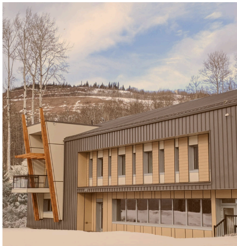
Figure 31. West Moberly First Nation Passive House Certified Health Centre by Iredale Architecture. Hildebrand, 2013.
