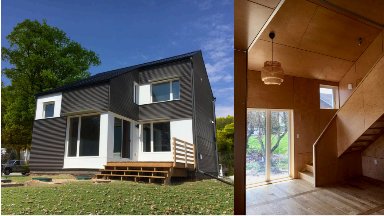
Figure 40. Exterior and interior photos of the Zero House completely assembled. Endeavour Center and Ryerson University, 2017.
