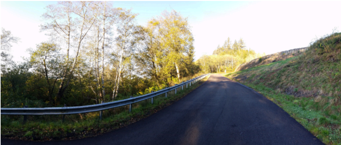
Figure 9. Eagle Hill Road Post-Construction, leading to the uplands. Red Plains Professional Inc., 2024.
