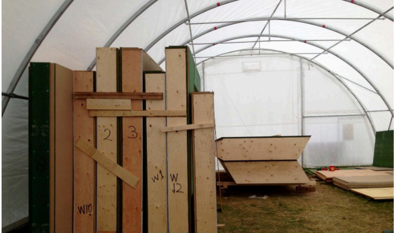
Figure 42. Storage of wall and roof panels, labeled and organized, inside the “Flying Factory” workspace. Endeavour Center and Ryerson University, 2017.
