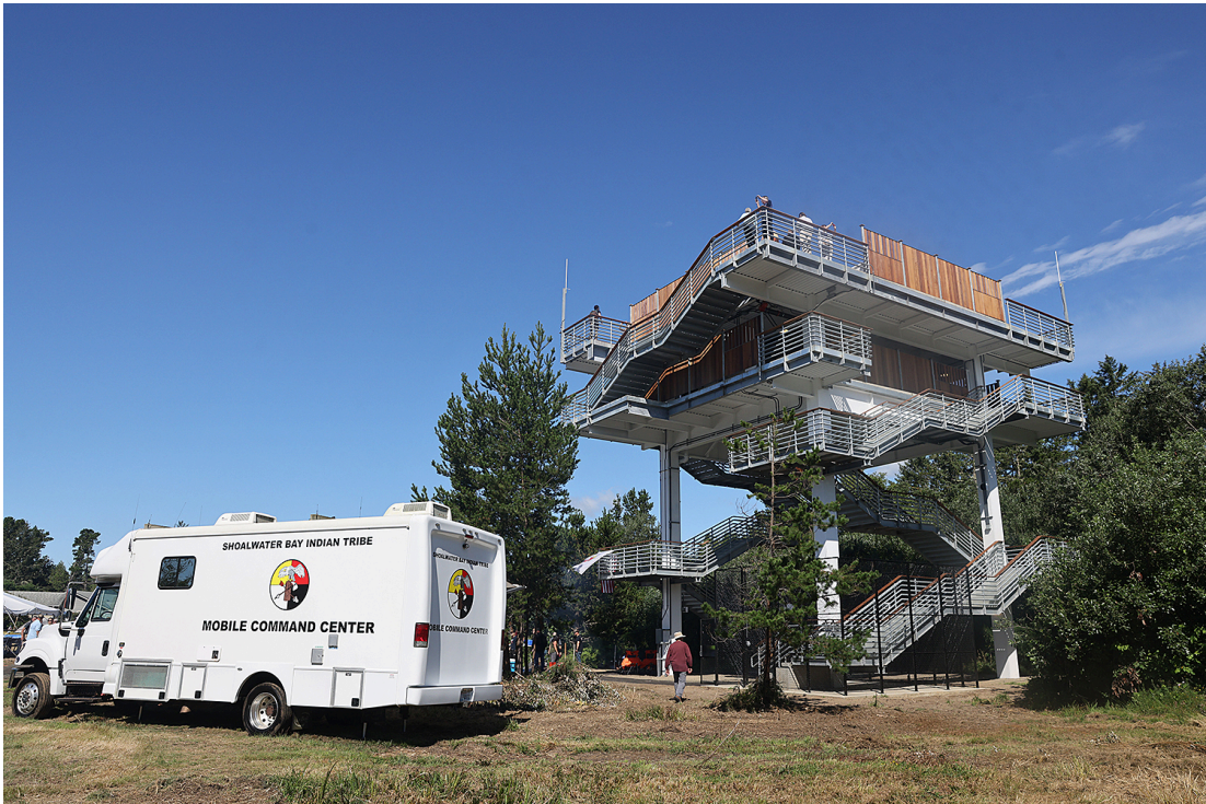
Figure 7. Shoalwater Bay Indian Tribe's Vertical Tsunami Evacuation Tower. WA Military Administrator, 2022.
