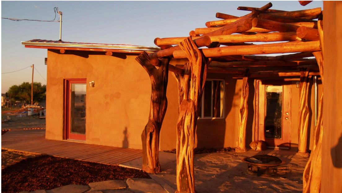
Figure 15. Nageezi House exterior includes reclaimed and gathered materials, and Navajo Flexcrete made from fly ash, 2005.
