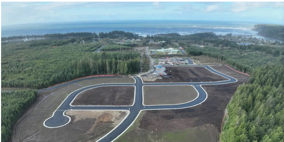
Figure 12. Progress of new village site, awaiting housing construction. Quinault Indian Nation Division of Natural Resources, 2023.
