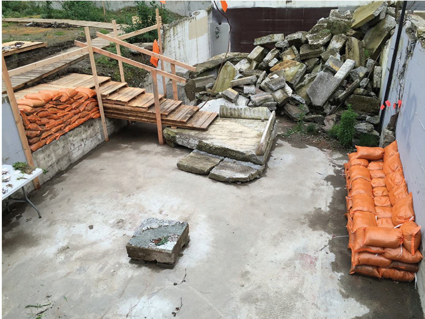
Demolition rubble rearranged to make foundation ruins into gallery space.
