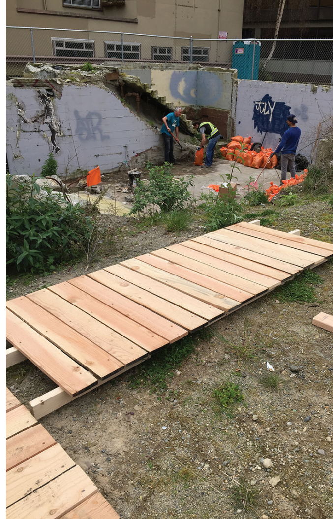
Boardwalk sections were prepared in advance and assembled on site.
