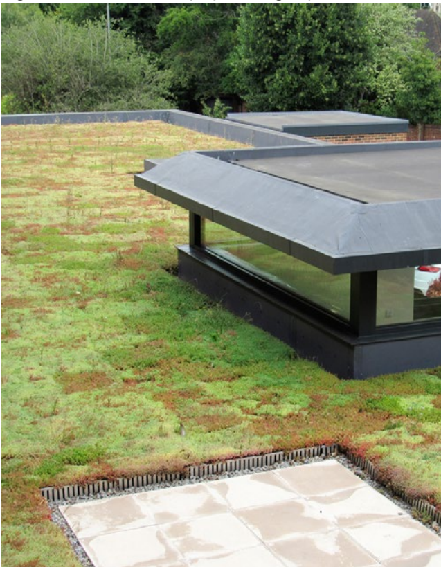
Figure 93. Sedum Rooftop by Roofing Superstore
