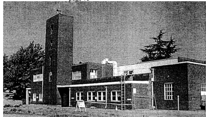
Figure 34. South side of the building. Source :Sand Point Magnuson Park Building 18 Firehouse Studio Project Feasibility Study Report By Arc Architects, page 1
