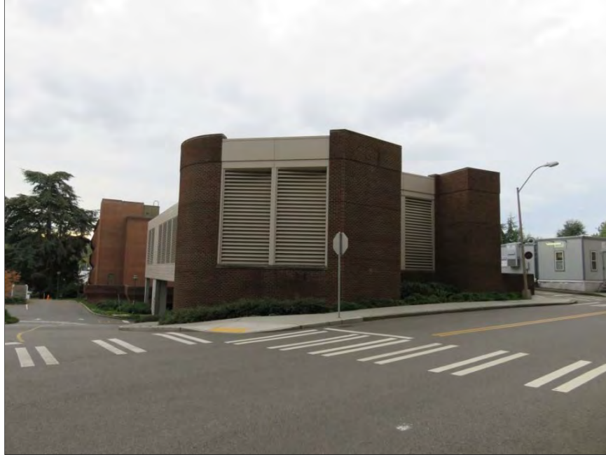
Figure 8-81. Eastern approach to South Campus Parking Garage, view southwest.
