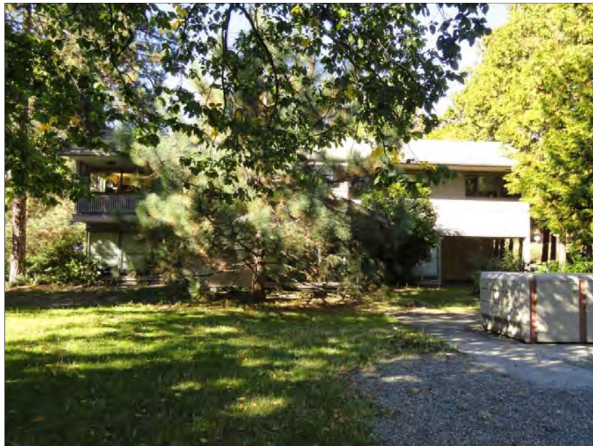
Figure 8-15. The south elevation of Guthrie Annex 3 with brick chimney and covered balcony, view north.
