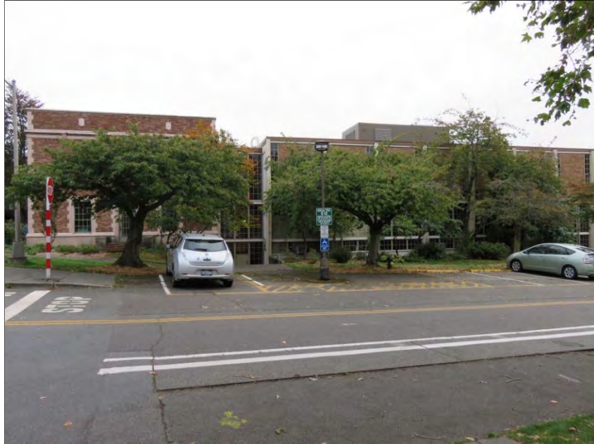
Figure 8-67. The west elevation of the Harris Hydraulics Laboratory, view east.
