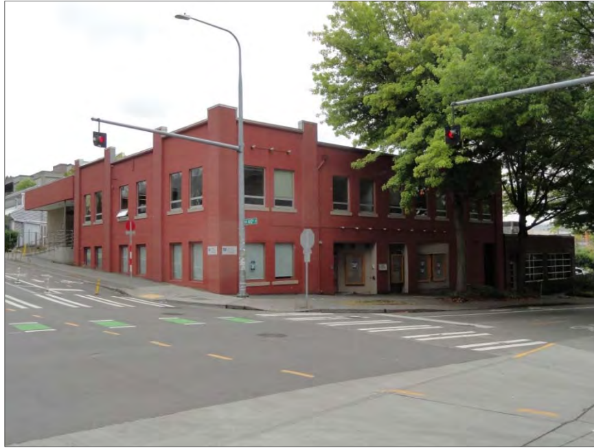
Figure 8-56. Northwest corner of 3930/3940 Brooklyn Ave. NE, view southeast.
