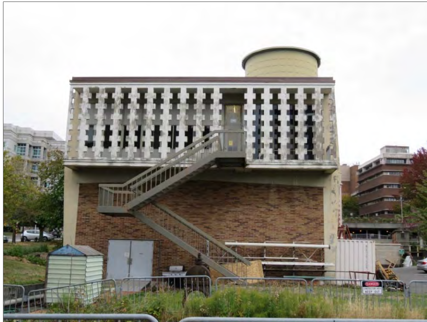
Figure 8-66. The south elevation of the Harris Hydraulics Laboratory, view north.
