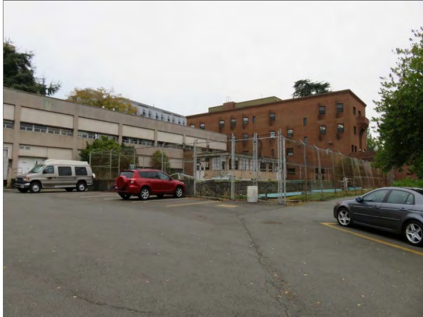
Figure 8-74. South elevation of the Portage Bay Building with fish ponds and 1969 addition.
