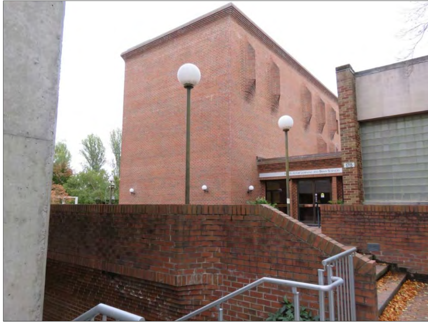
Figure 8-75. Primary north entrance to the Portage Bay Building addition, view southeast.
