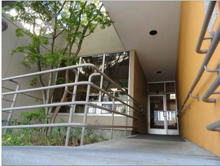
Figure 8-58. Detail of entry, addition on 3930 Brooklyn Ave. NE, view south.
