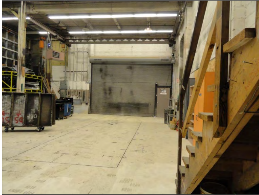
Figure 8-45. Interior of shop, 3939 University Way NE, view west.
