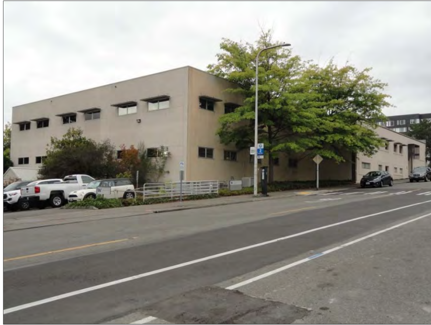
Figure 8-31. 3917 University Way NE, original building plus 1980 addition, view northeast.
