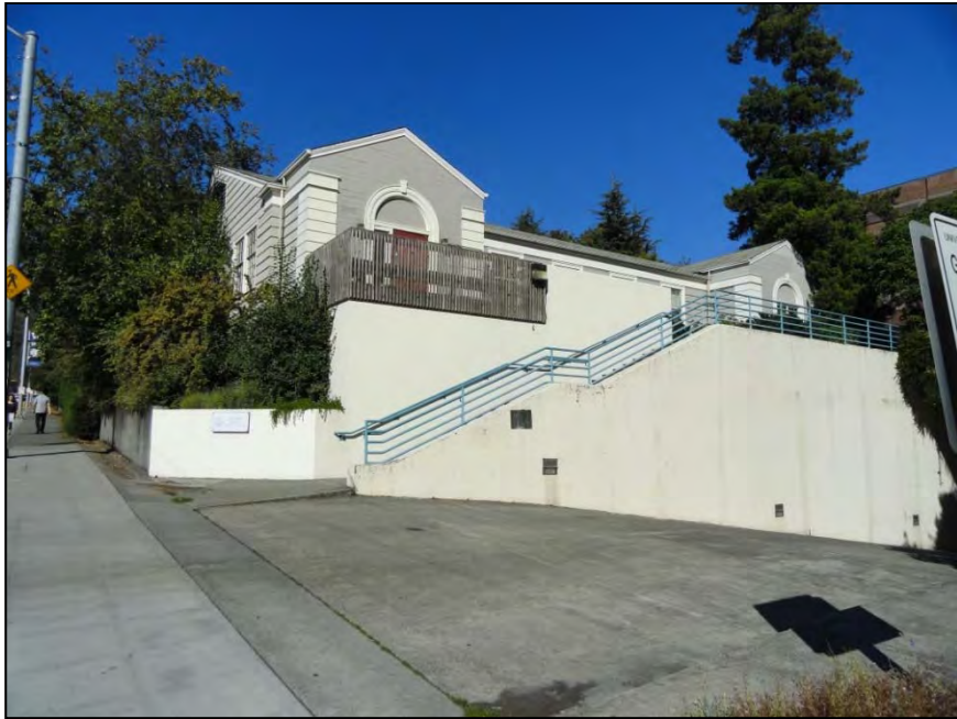
Figure 8-4. South elevation of Guthrie Annex 1 with retaining wall, view north.
