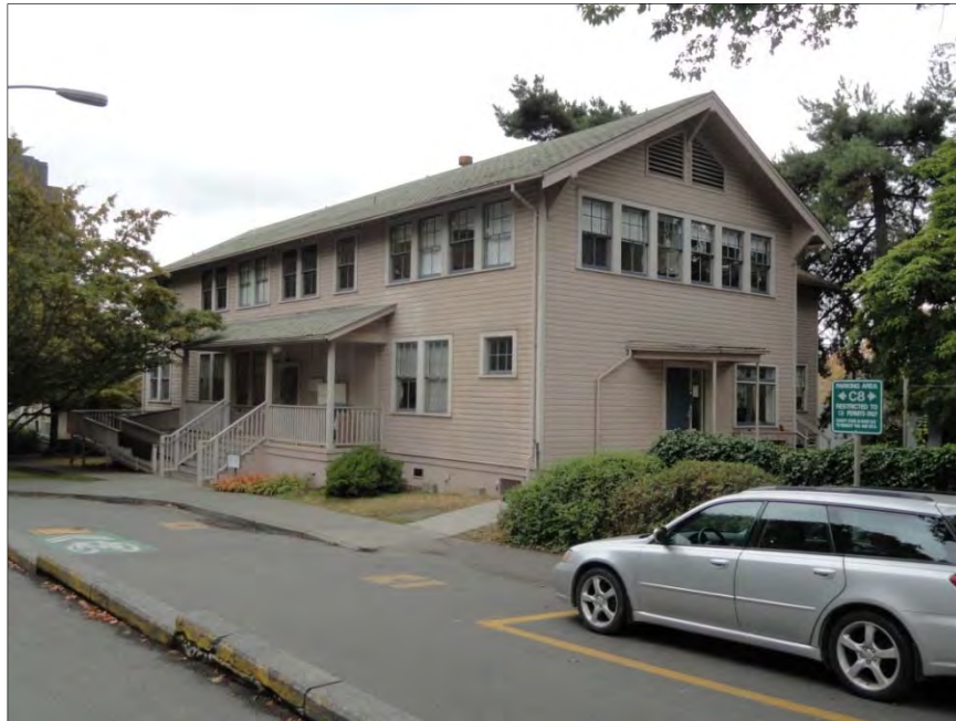
Figure 8-9. Guthrie Annex 2, view southwest.
