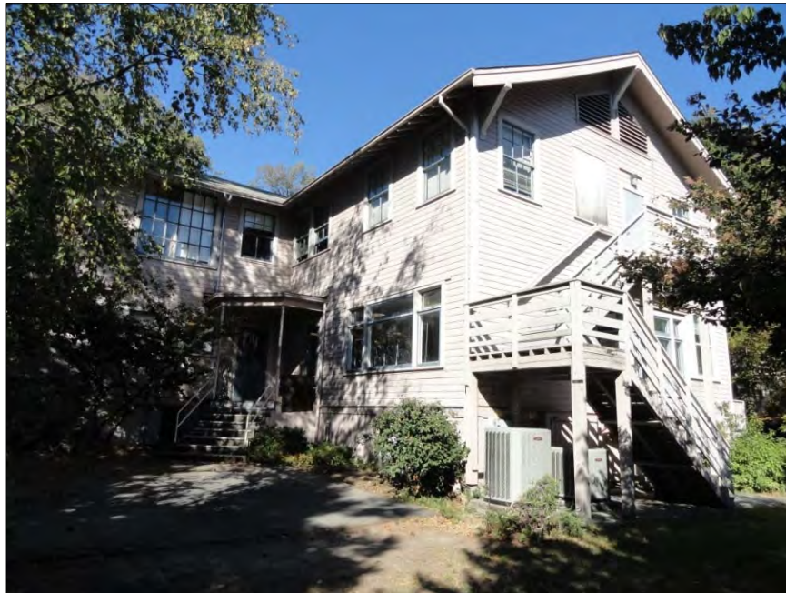
Figure 8-11. South elevation of Guthrie Annex 2, view northeast.
