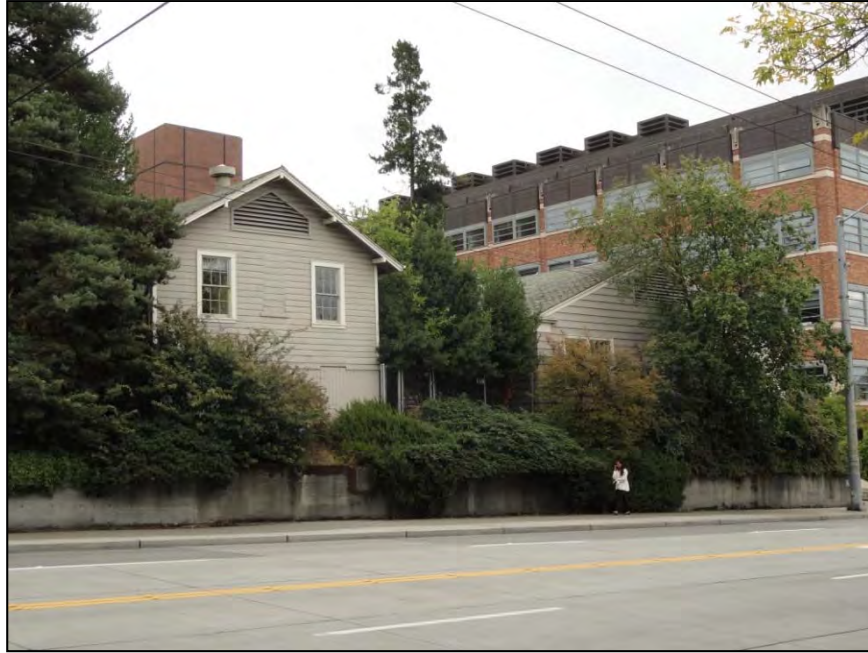
Figure 8-5. West elevation of Guthrie Annex 1, north and south wings, view east.
