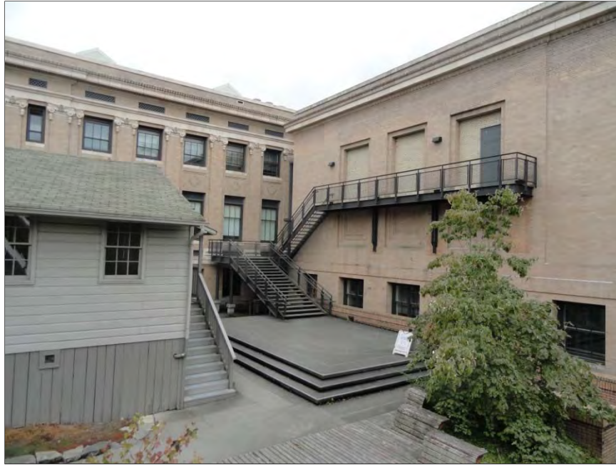
Figure 8-29. The south elevation of Architecture Hall, view east.
