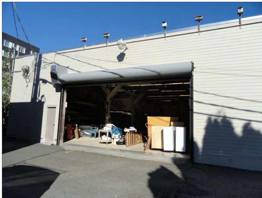
Figure 8-50. West elevation of 3941 University Way NE, view east.
