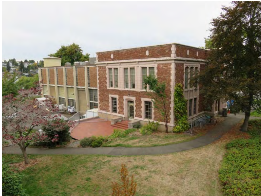
Figure 8-65. The Harris Hydraulics Laboratory and its addition, view west.
