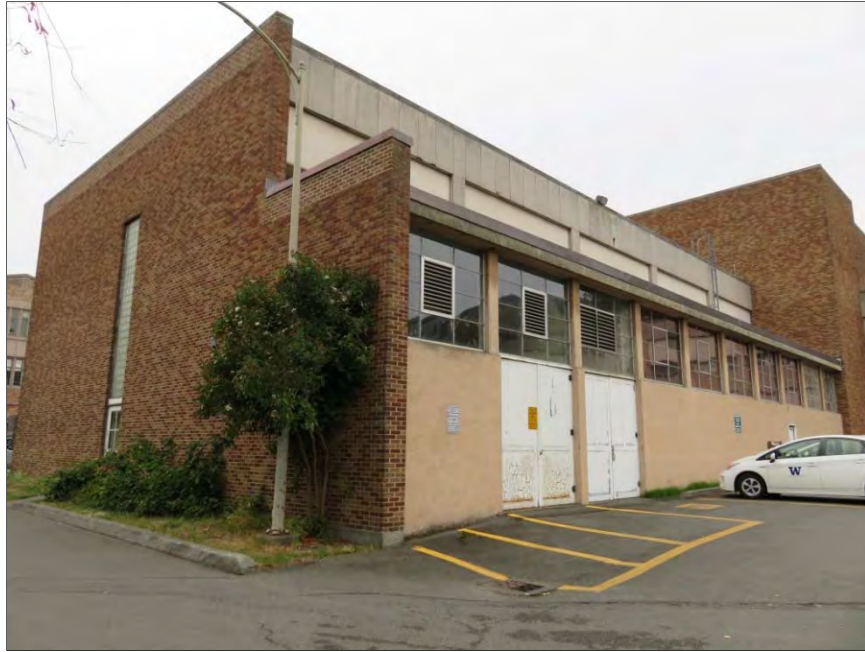
Figure 8-73. West wing of the Portage Bay Building, view northwest.
