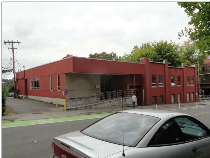
Figure 8-57. 3930 Brooklyn Ave. NE with 1980s addition, view south.
