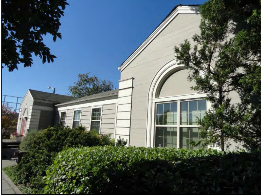
Figure 8-3. The south elevation of the south wing of Guthrie Annex 1, view northwest.
