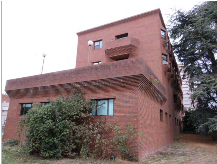
Figure 8-76. Portage Bay Building addition, view northwest.
