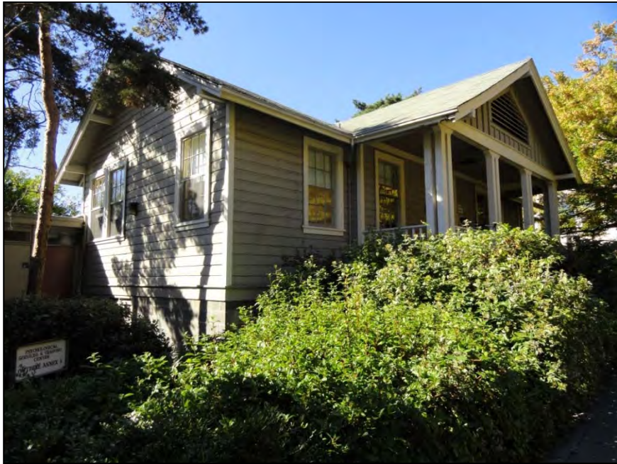
Figure 8-2. The north wing of Guthrie Annex 1, view northwest.
