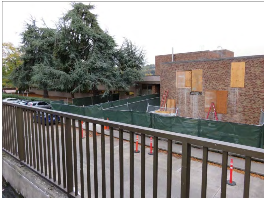
Figure 8-72. North façade of the Portage Bay Building, view southwest.
