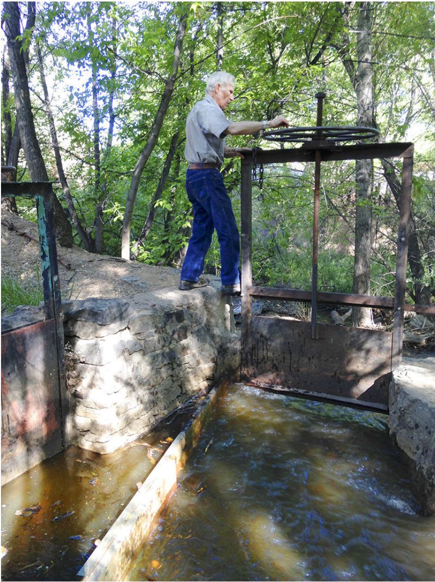
Figure 28: Parciante opening a headgate
