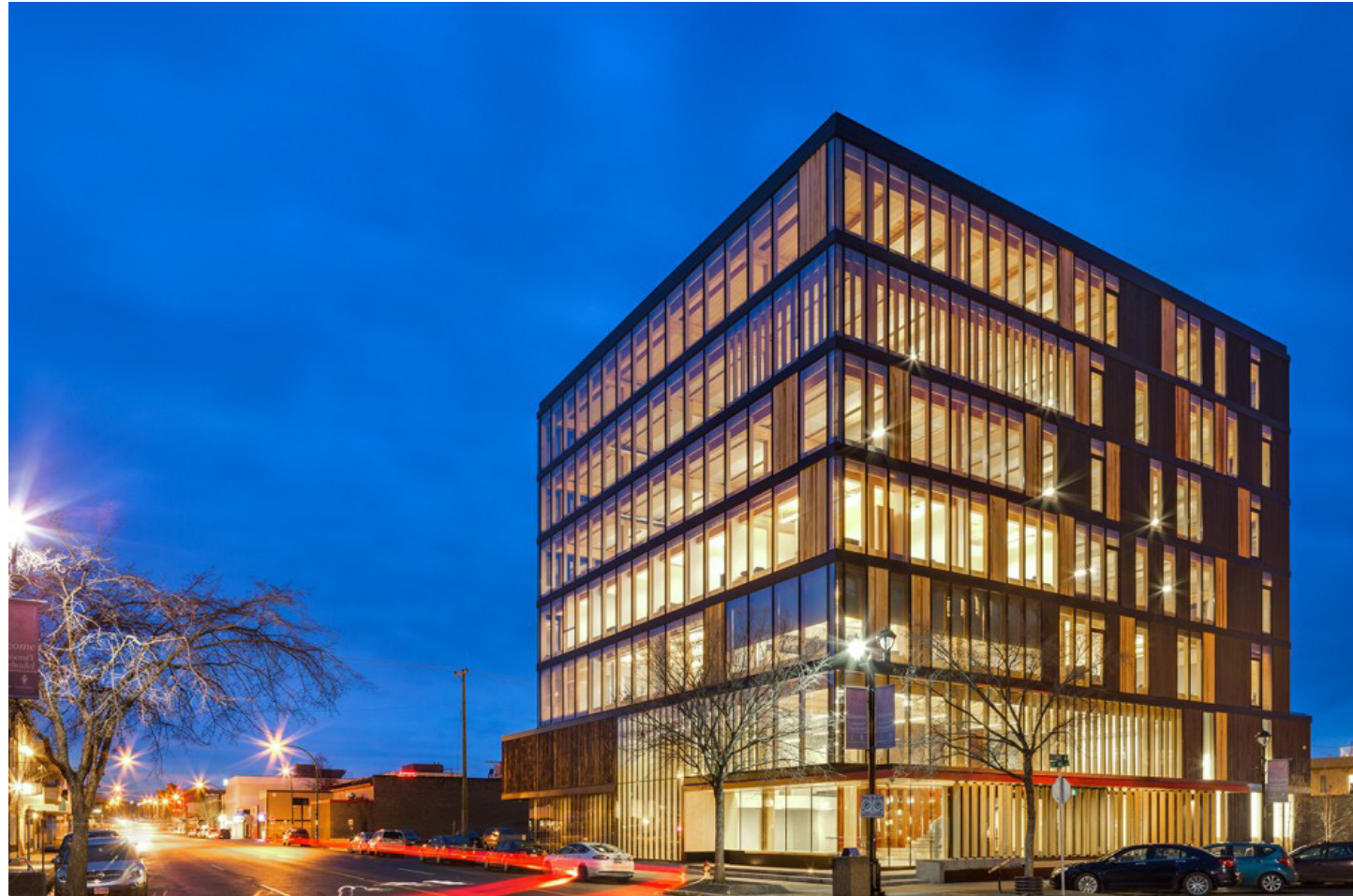
Figure 45. Wood Innovation and Design Center (from Michael Green Architecture)
