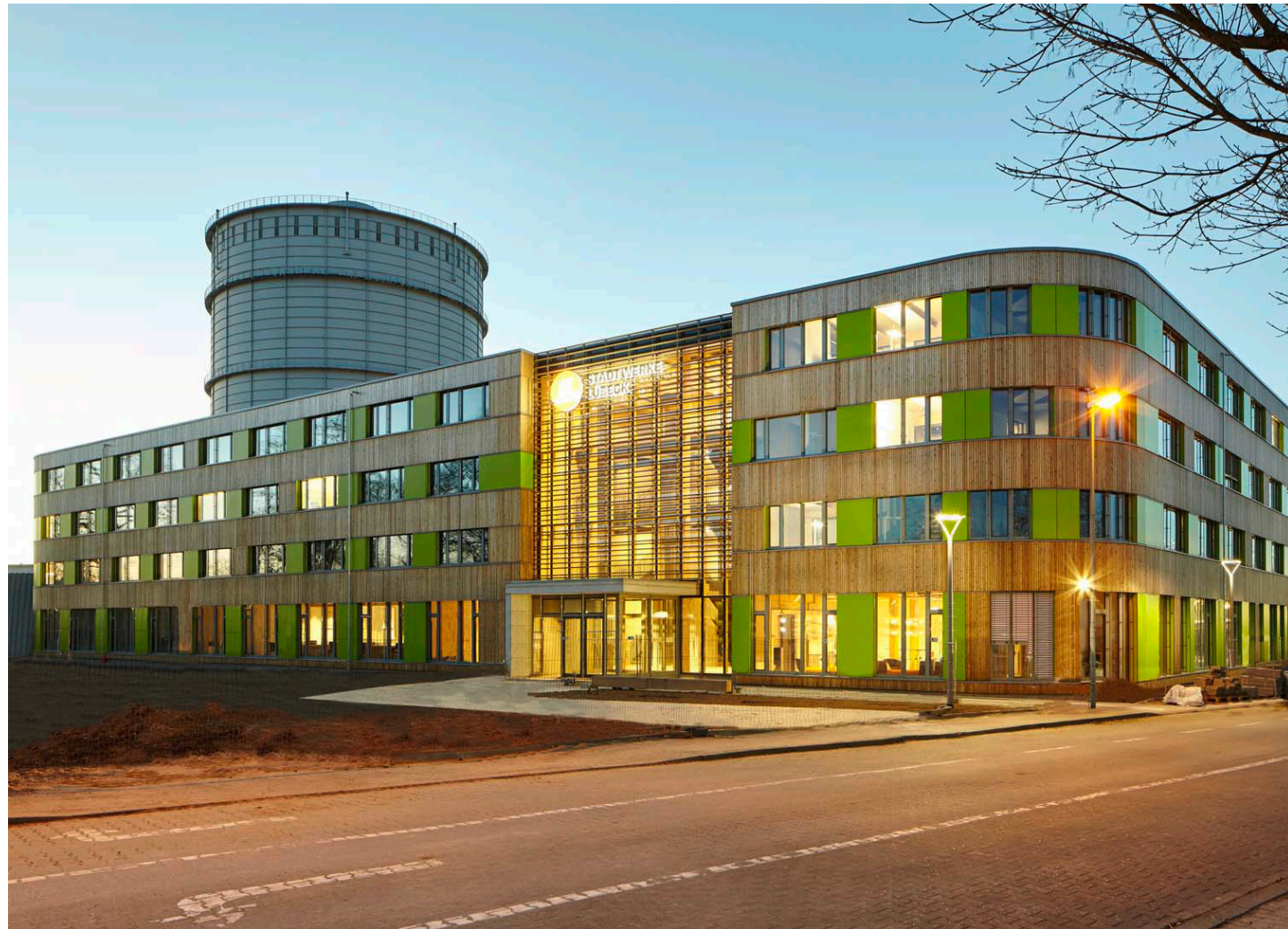
Figure 49. Stadtwerke Lübeck Headquarters (from FpbrAG)
