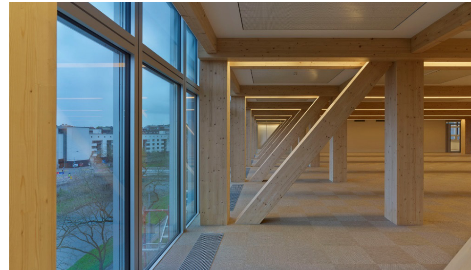
Figure 61. View of Structure (Top) (from Shigeru Ban Architects)
