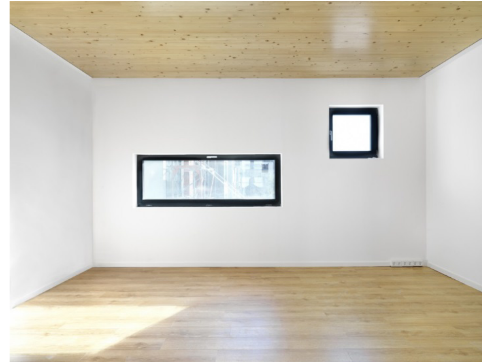
Figure 66. Exposed CLT in Finished Structure (Left) (from Kaden Klingbeil)
