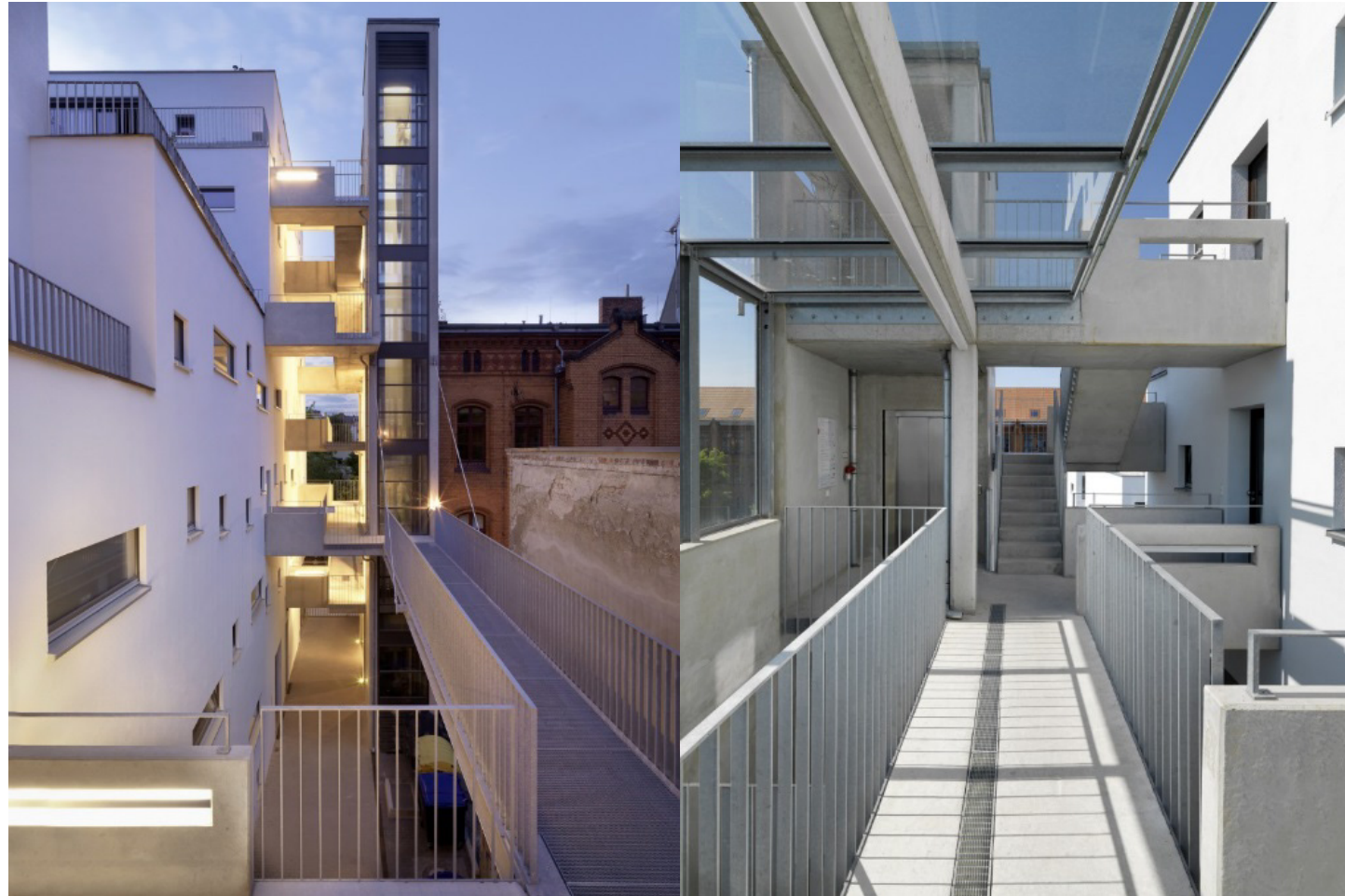
Figure 64. C13 Building (Left) (from Kaden Klingbeil)
