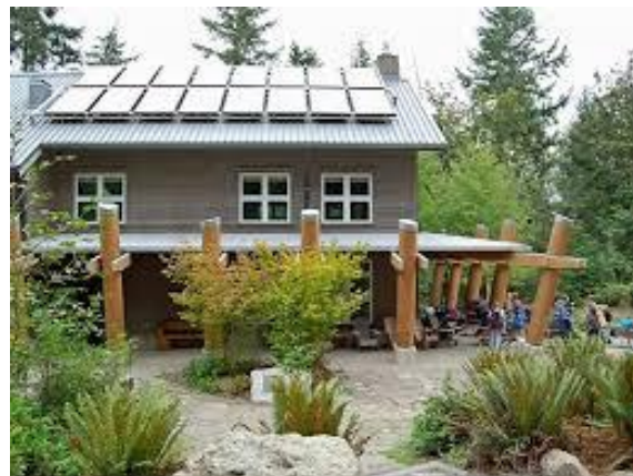
Figure 17. Ecologically low-impact stormwater- and draught-tolerant environmental educational retreat at Islandwood, Bainbridge Island (Berger Partnership)
