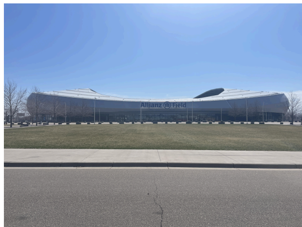
Figure 10: Current Allianz Field Photo
