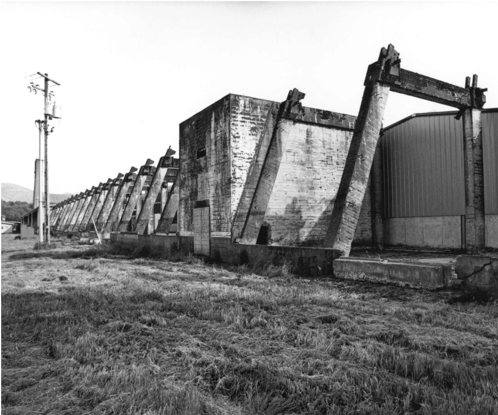
figure 71 tillamook hangar a ruins 2014
