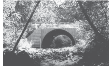
Arch culvert in the Soos Creek watershed.
