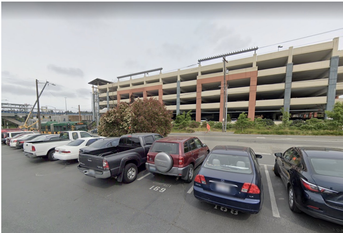
Figure 27: Ground Parking and Parking Garage near Northgate Transit Center
