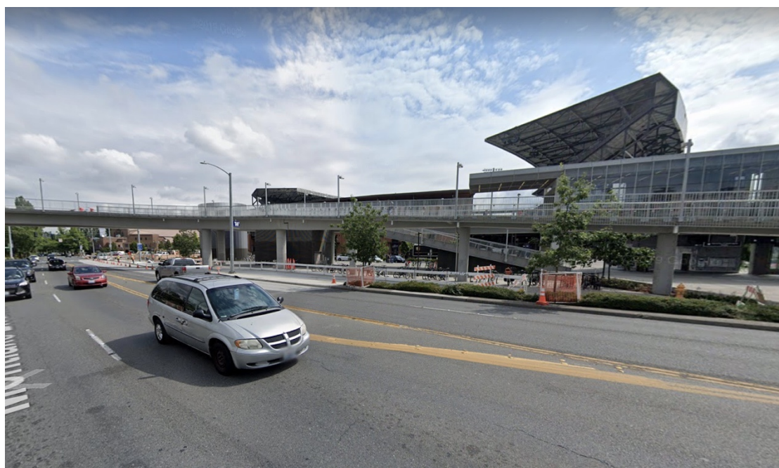
Figure 28: Pedestrian Bridge Over Montlake Boulevard at the University of Washington Light Rail Station
