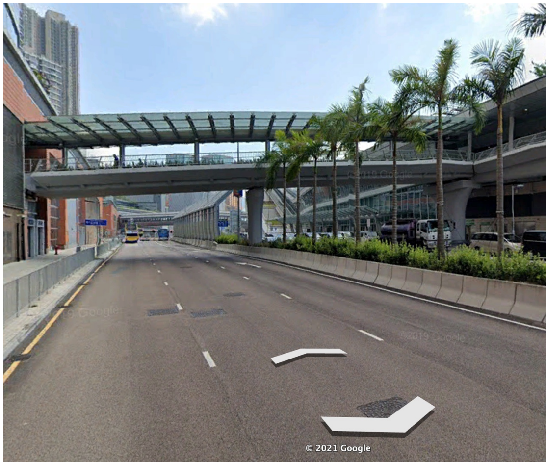
Figure 12: Wui Man Road View (Next to Kowloon transit center)
