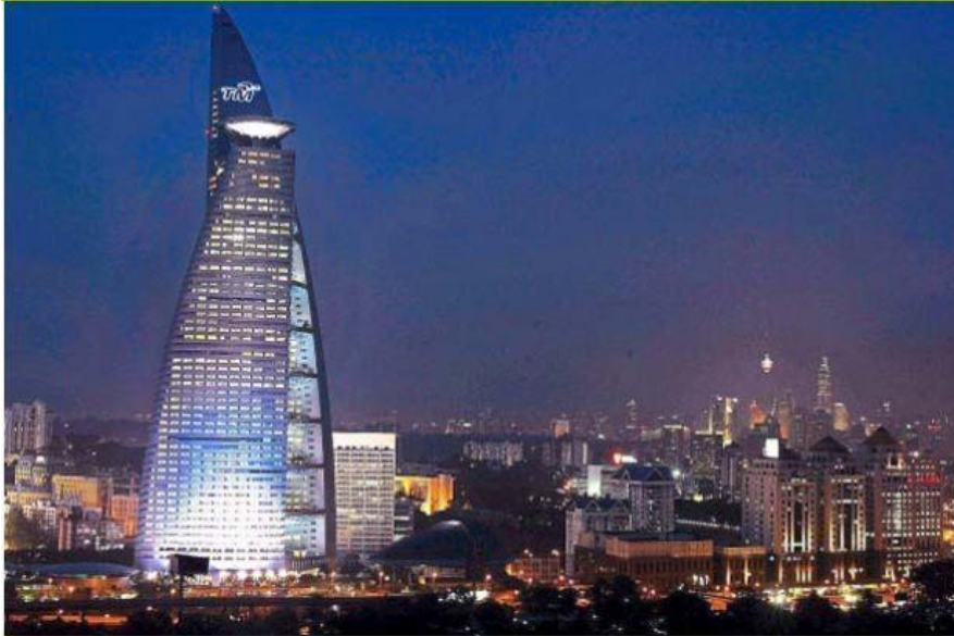
Figure 4: Telekom Malaysia communications tower. Accessed 20 February 2017. Photo courtesy of The Star Online < http://www.thestar.com/my/business/business-news/2015/12/18/tm-to-invest-rm23bil/ >.
