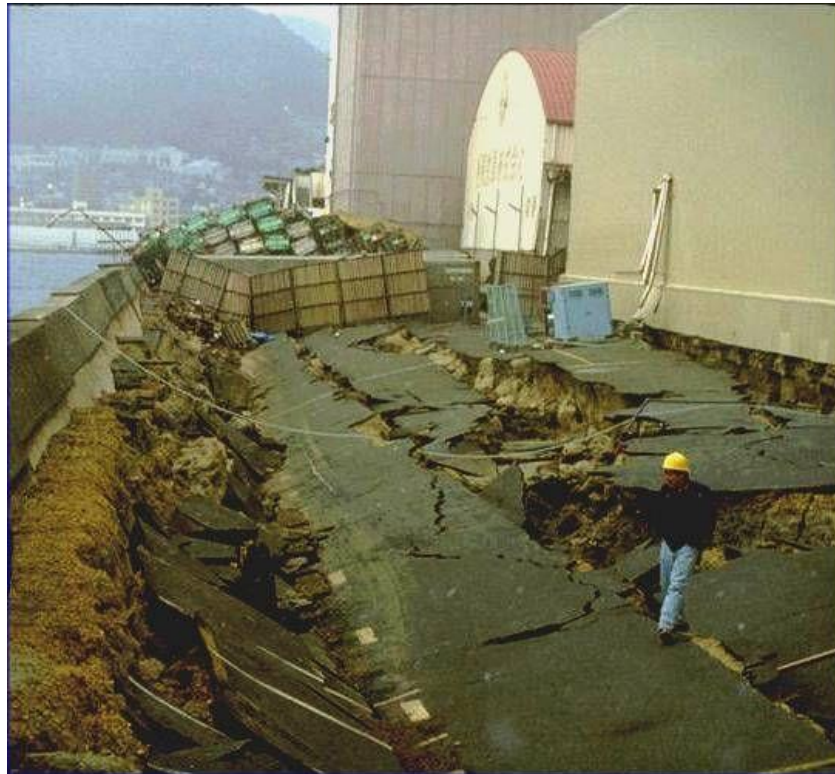
Figure 5.2. Liquefaction-induced lateral spreading from the 1995 Kobe, Japan earthquake causing severe damage to a quay wall (UW).
