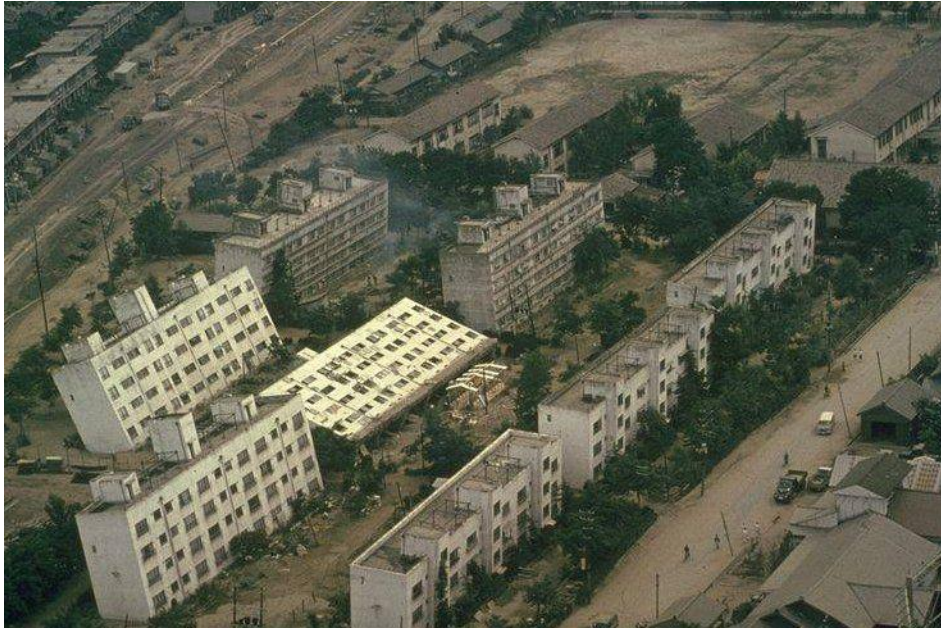
Figure 2.1. Bearing capacity failure of the Kawagishi-cho apartment buildings due to flow liquefaction (USGS).
