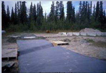
Spanning 12 foot void
