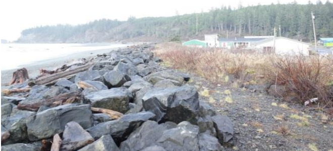
Figure 7. The existing Seawall in Taholah. Storm surges have recently surpassed this barrier.
