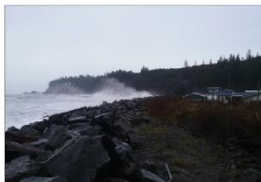
Seawall to protect the village of Taholah, WA from storm surges.
