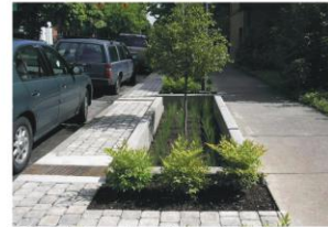
Simple features like this one in Portland, Oregon are a cost-effective and attractive way of collecting stormwater runoff using native plantings.
