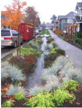
Figure 13. Bioswale at High Point. Source: SvR Design.
