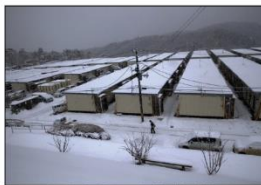
Temporary housing for thousands of families in Minamisanriku, Japan.
