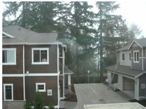
Figure 15. Shared Driveway at Sycamour Park. Photograph taken by the author.
