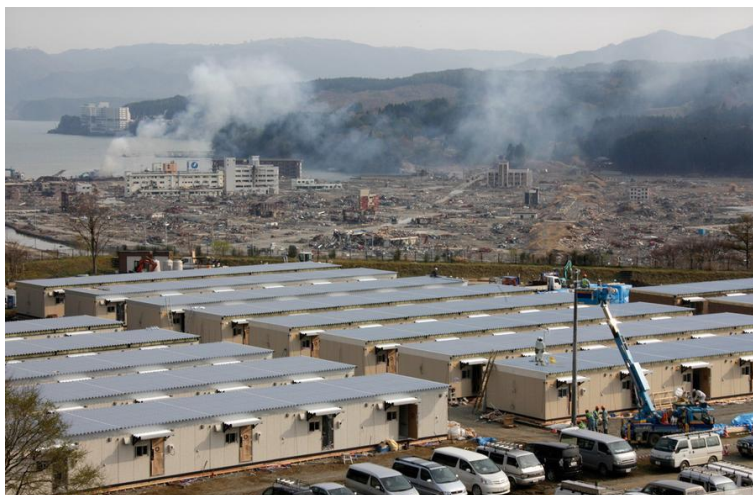
Figure 4. Temporary Housing Outside of Disaster Zone in Minamisanriku, Japan. Source: The Atlantic.
