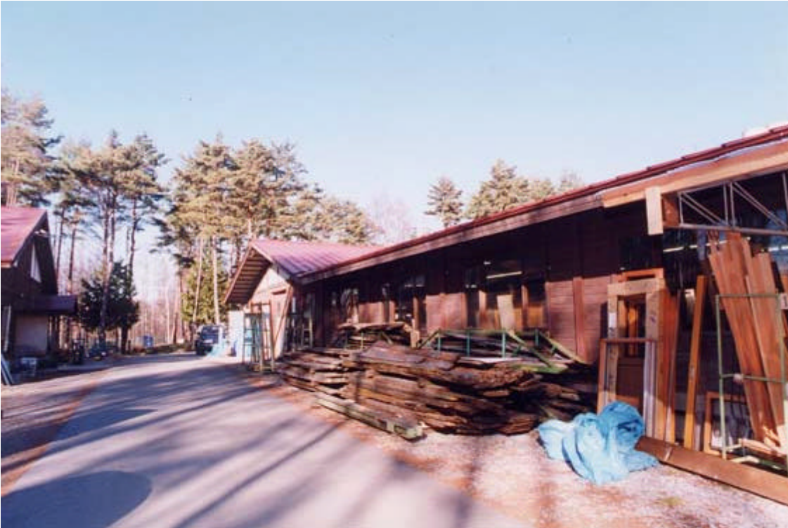
Figure 21. A small wooden window manufacturer located in Chino City, Nagano prefecture.
