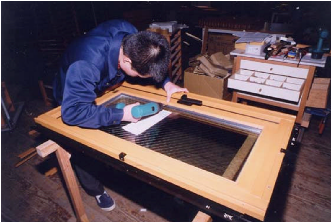
Figure 24. Worker installing a glass pane in a window.
