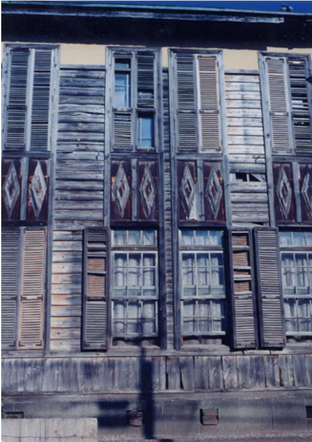
Traditional Japanese wooden windows and shutters provide an interesting exterior pattern on older Japanese post and beam homes.
