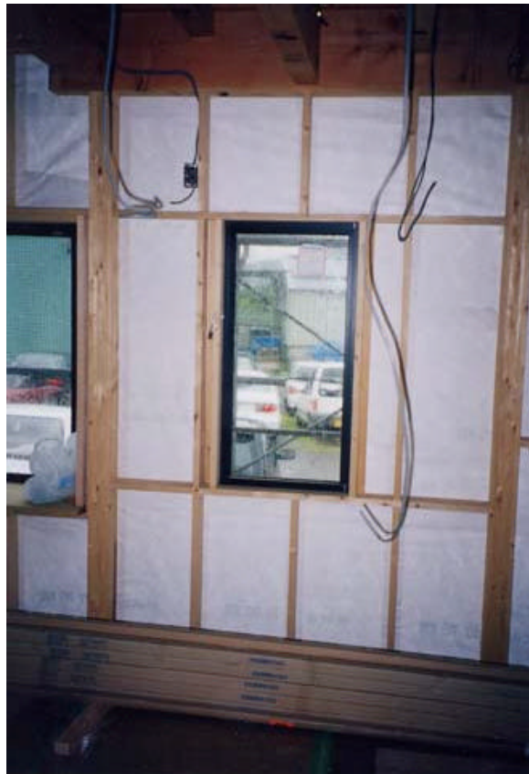
Figure 38. Windows are often framed in between the structural posts in Japan.
