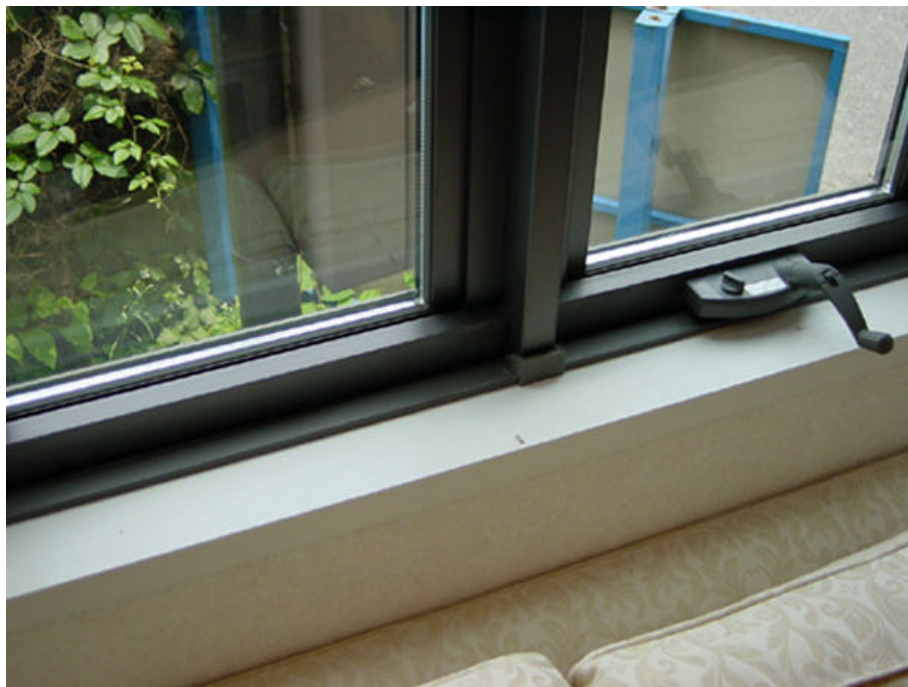
Figure 48. Removable joint strip covers the small gap where the sash butts up to the window. Note that the interior sill of the window is white plastic lumber with a wood grain impression.
