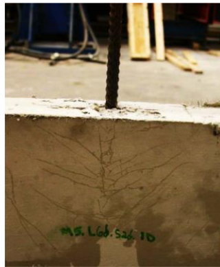
Figure 7.5. Diagonal crack pattern observed by Graybeal.
