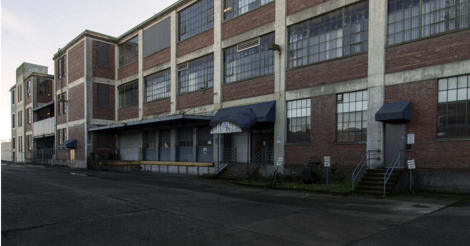
fig. 11: Industrial building that is currently used for recycling - adaptable framework
