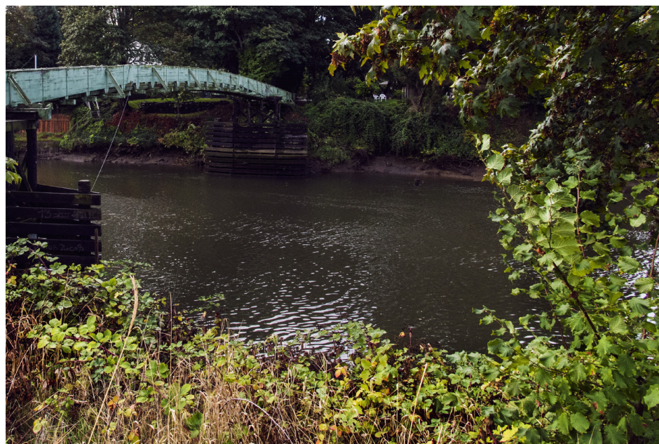
fig. 15: Pedestrian Bridge over the Duwamish River in Tukwila
