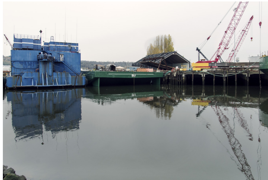
fig. 14: Barges docked along Slip 4 in the Duwamish Waterway
