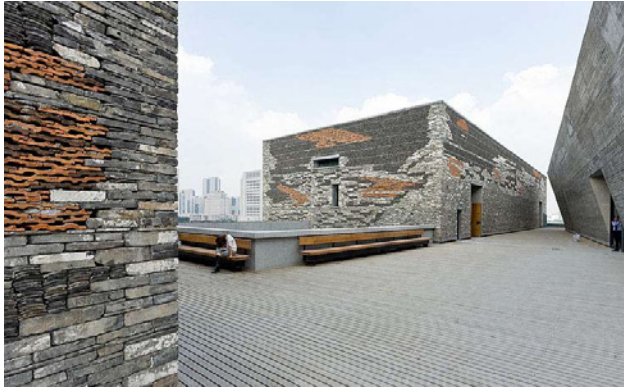
Fig. 2.4 Ningbo Historic Museum, Ningbo, China, Wang Shu
