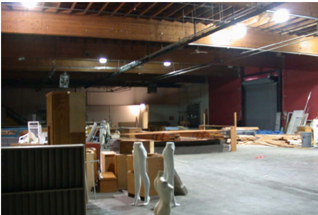
Fig. 3.10 Interior view of the existing SPU warehouse
