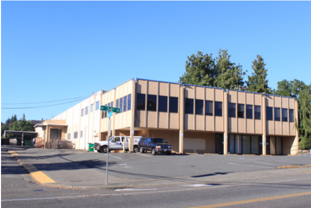
Fig. 3.9 Exterior view of the existing SPU warehouse
