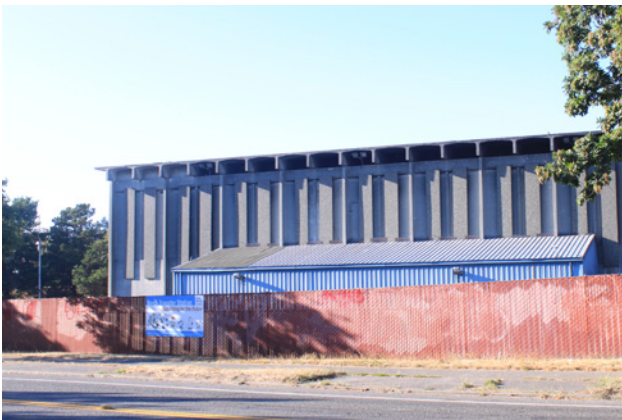
Fig. 3.1 Existing Seattle North Solid Waste Transfer Center
