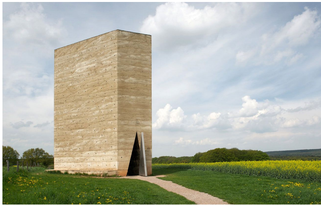
Figure 6. Bruder Klaus Field Chapel, Wanchendorf, Germany complete.
