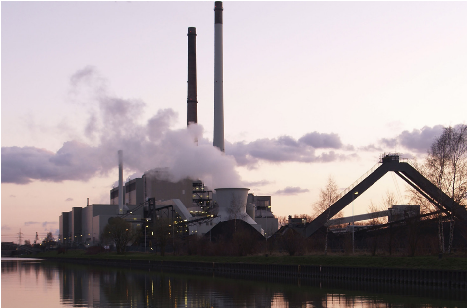
Figure 4. Coal fired Power Plant
