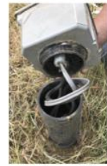
Lack of access: 15% Limited cable slack: 18%
