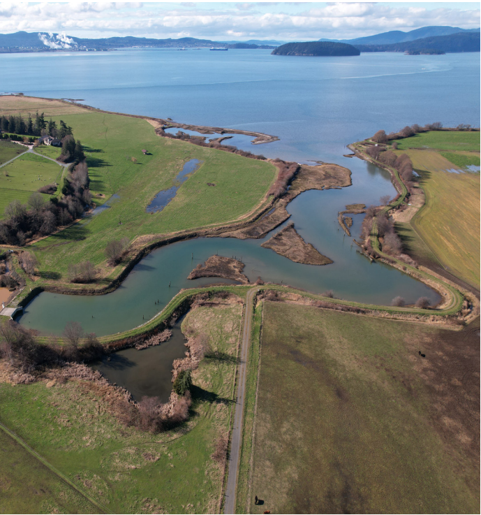
Figure 3.6: Drone photograph of Joe Leary Slough at Padilla Bay. Image by author.
